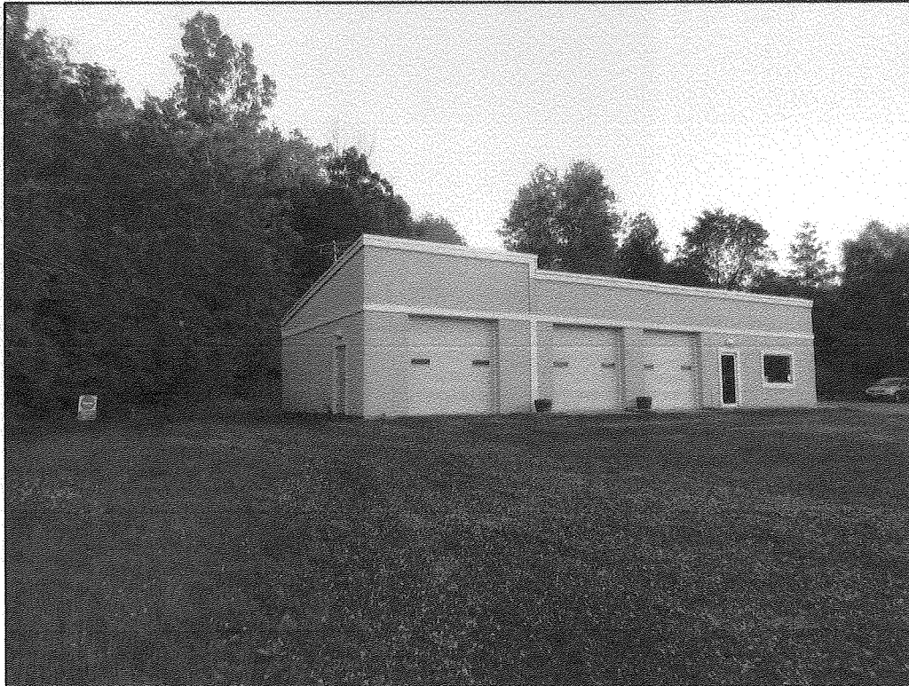
PICTURE # 2 NORTHEAST PROPERTY FRONTAGE ALONG SOUTH PLANK ROAD
