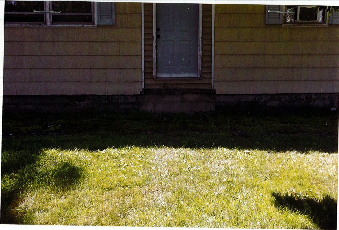
FRONT VIEW LOOKING WEST
