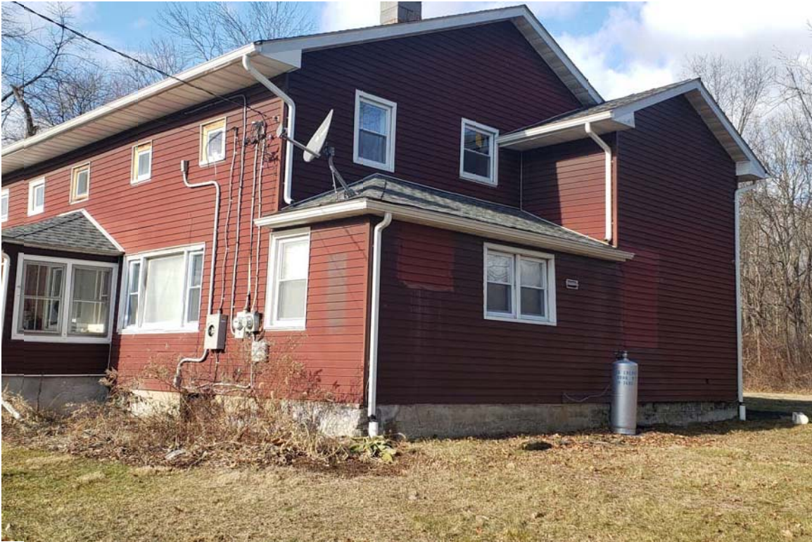
FIGURE 7: SOUTHEAST CORNER OF RESIDENCE
