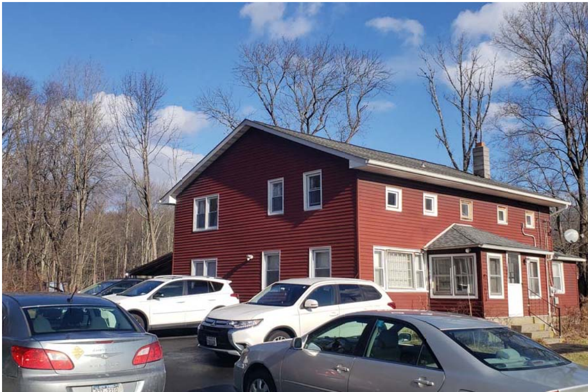
FIGURE 2: LOOKING ACROSS DRIVEWAY AT SOUTHWEST CORNER OF RESIDENCE
