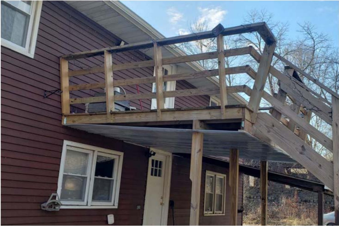
FIGURE 1: DECK ACCESS TO SECOND STORY UNIT
