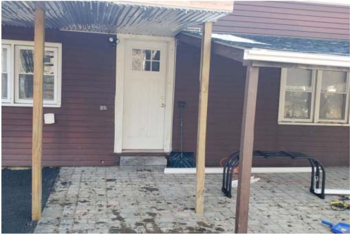
FIGURE 5: NORTH ACCESS TO GROUND FLOOR UNIT
