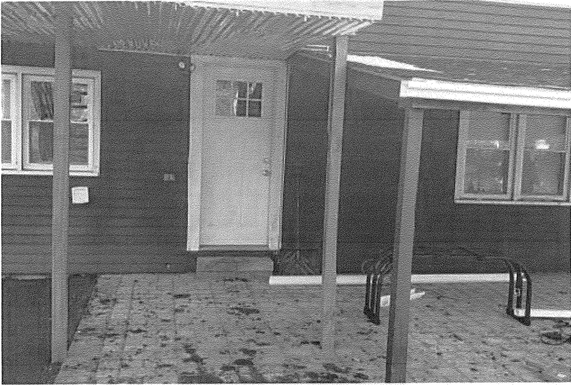
FIGURE 5: NORTH ACCESS TO GROUND FLOOR UNIT
