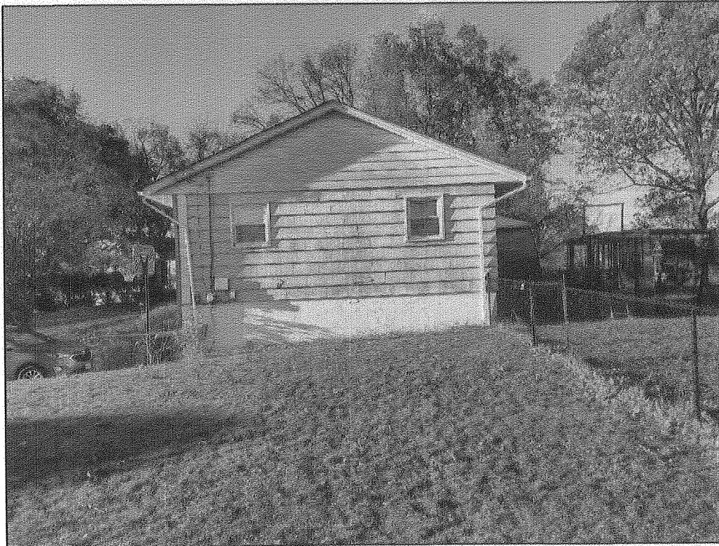
PICTURE # 2 RIGHT (SOUTH) SIDE ELEVATION
