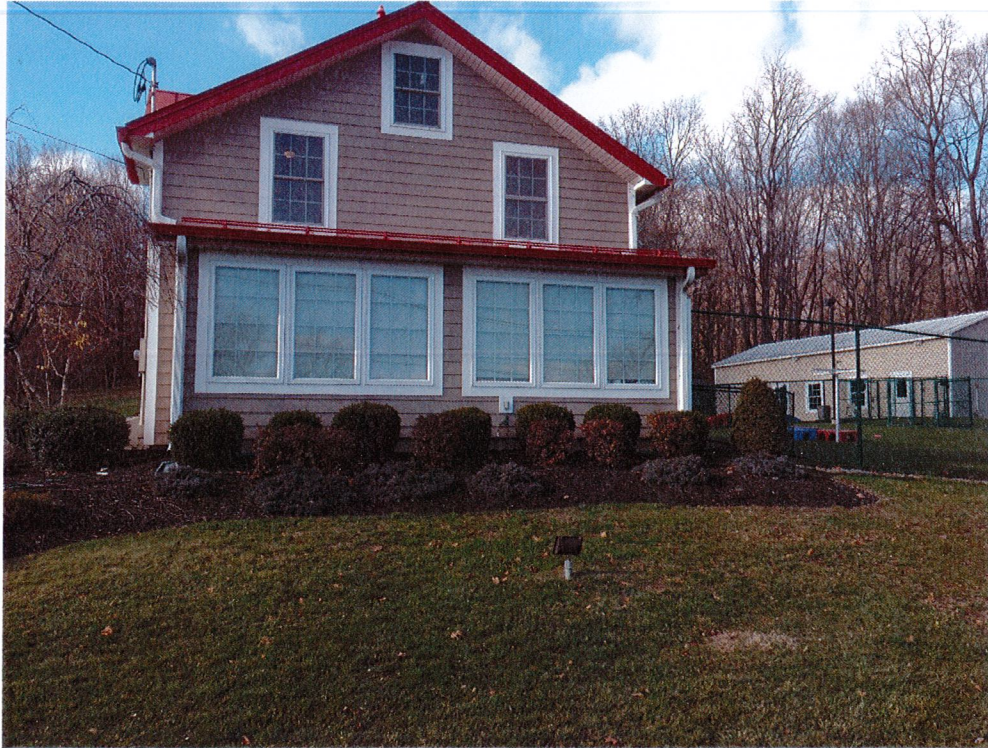
Front view of existing structure (East)
