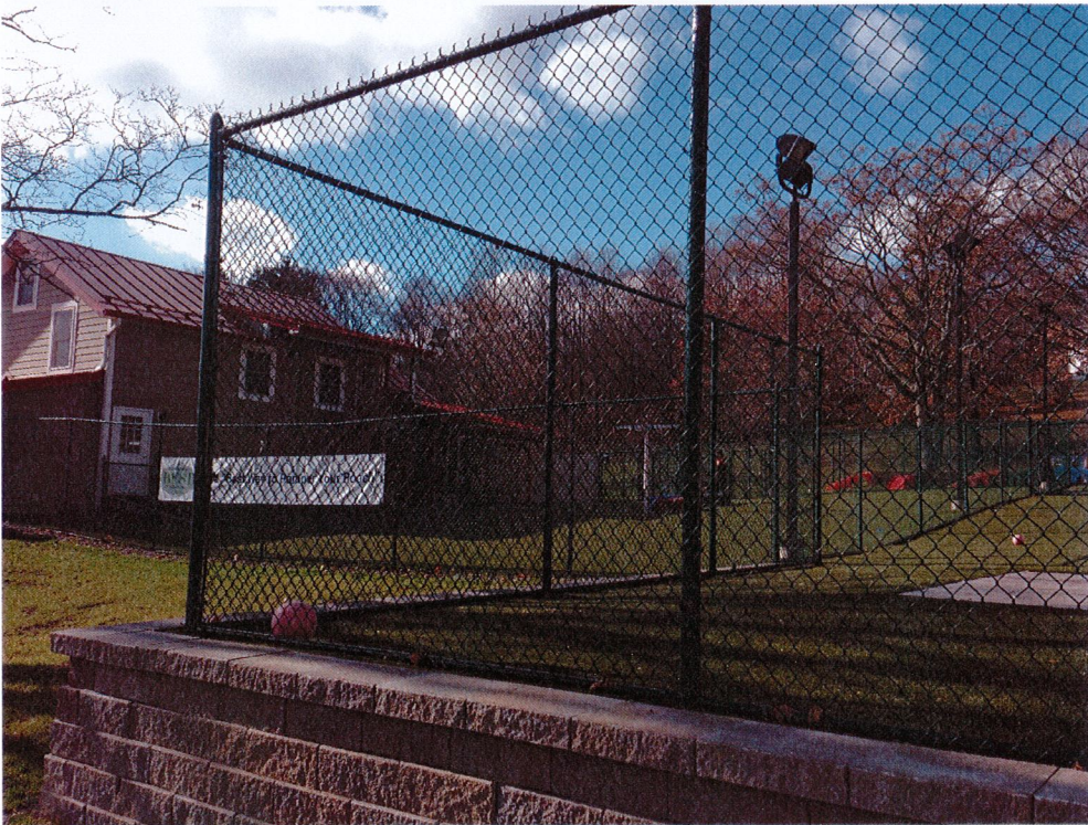
Side view of existing structure (North)
