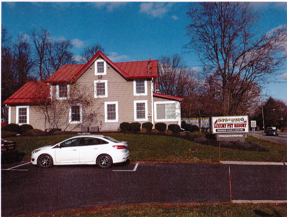
Side view of existing structure (South)
