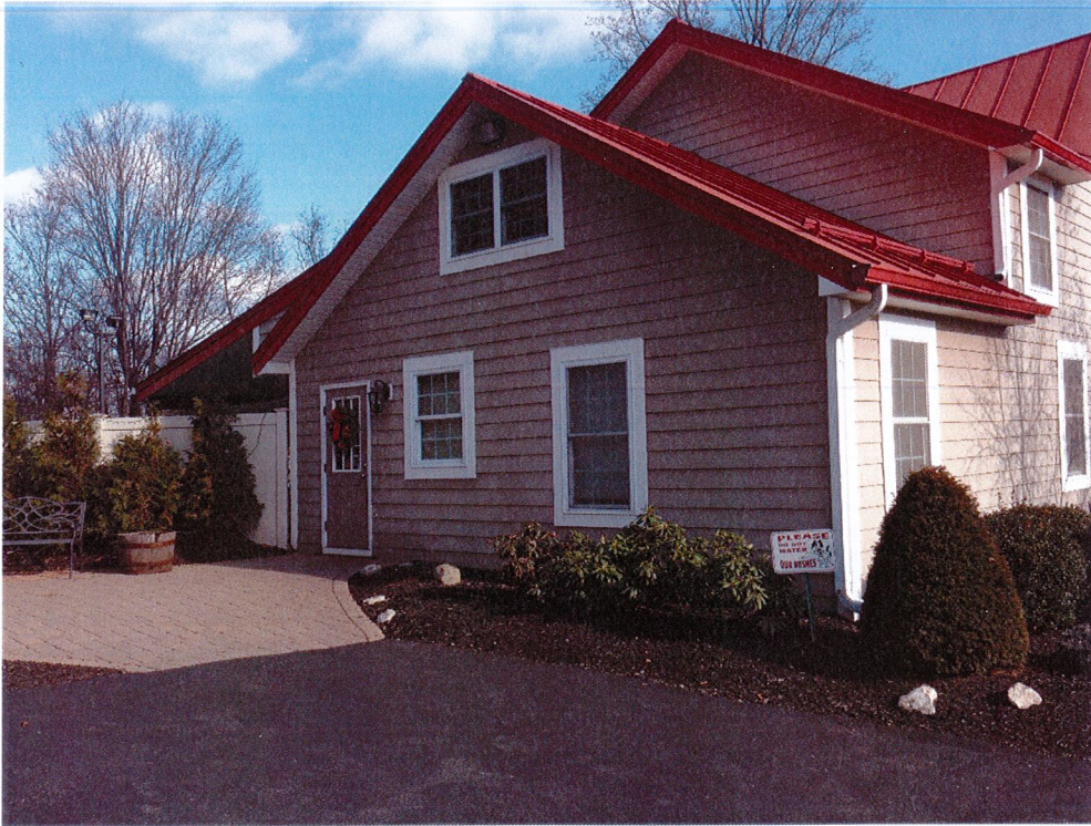
Rear view of existing structure (West)
