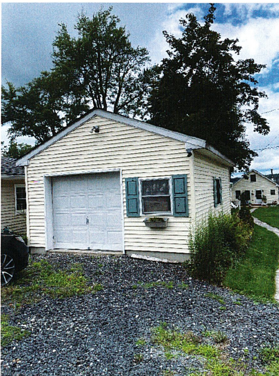
Garage- Front (East elevation)
