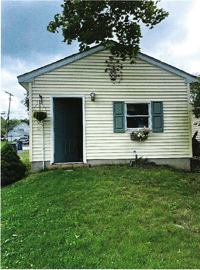
Garage- Rear (West Elevation)
