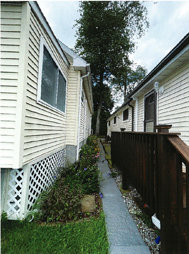
House - Left (South Elevation)
