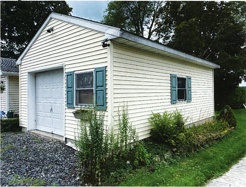
Garage – Right (North elevation)
