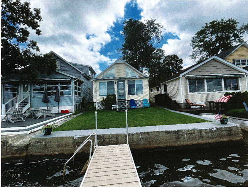
House- Rear ( West Elevation)
