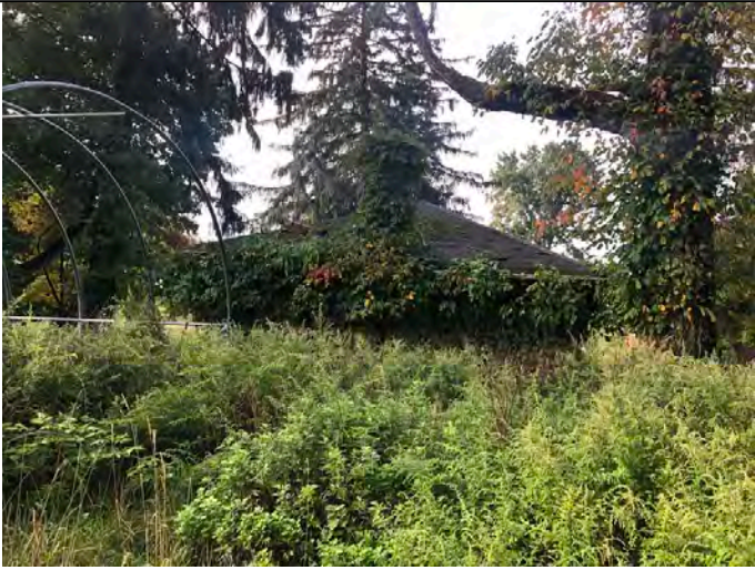
Site Building 2 north exterior
