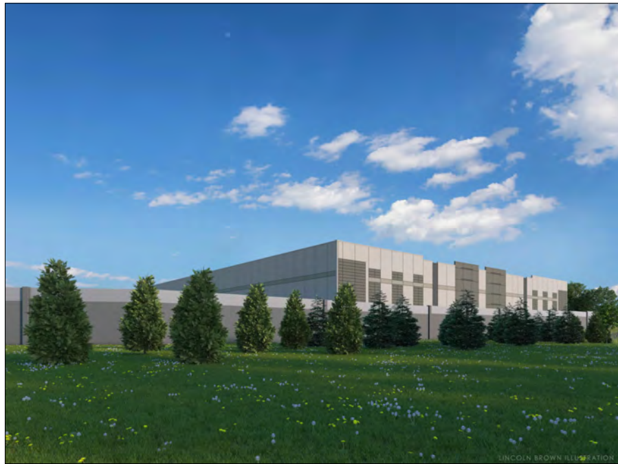
TIME OF PLANTING VIEW FROM 128 ROUTE 17K
