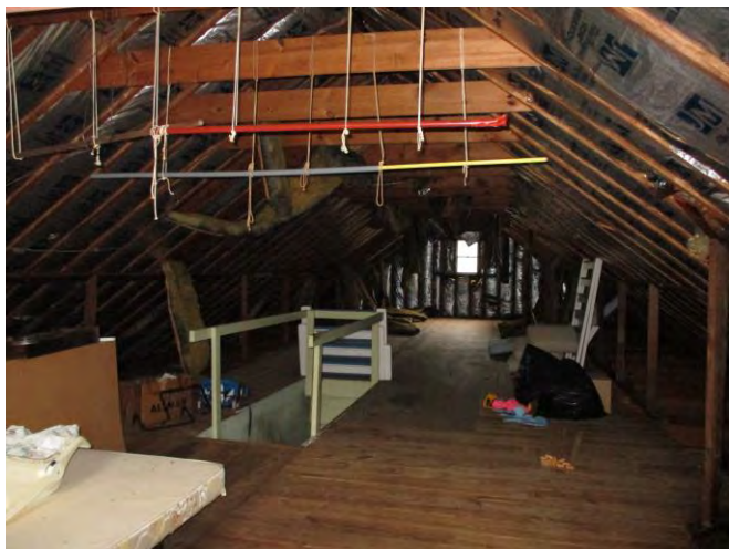
Photo 11 General View of Attic
