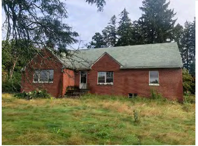
Site Building 1 south exterior
