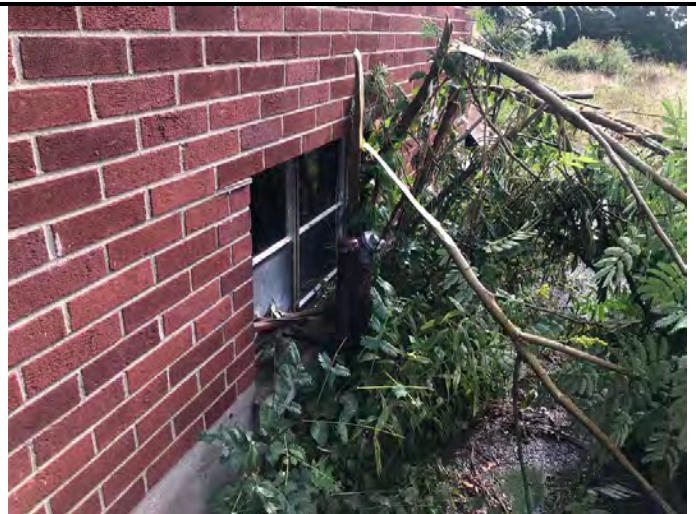
Site Building 1 fill and vent pipes
