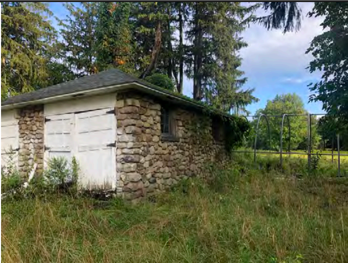
Site Building 2 east exterior
