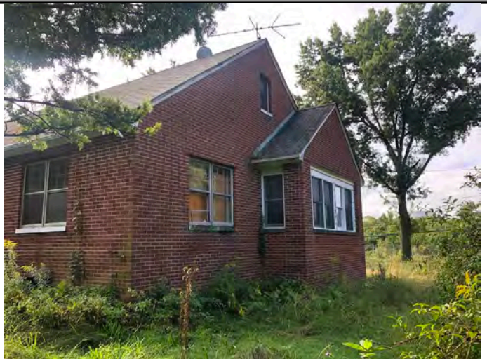
Site Building 1 west exterior
