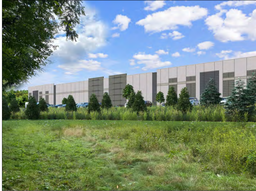
TIME OF PLANTING VIEW FROM 120 ROUTE 17K
