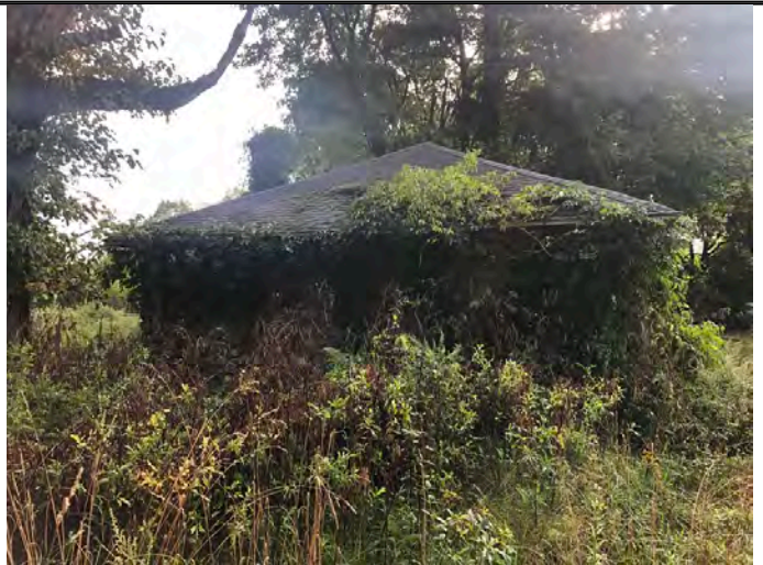
Site Building 2 west exterior
