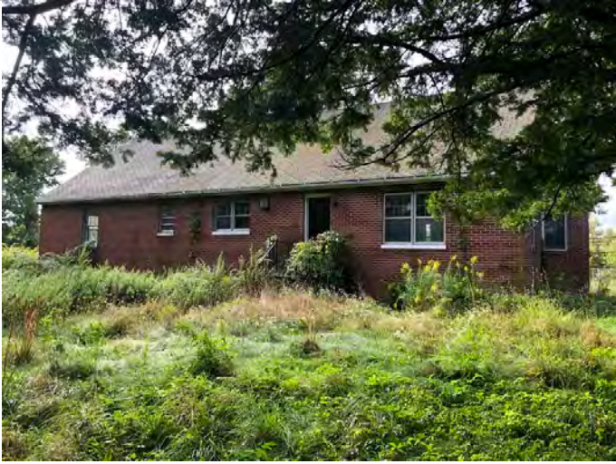
Site Building 1 north exterior
