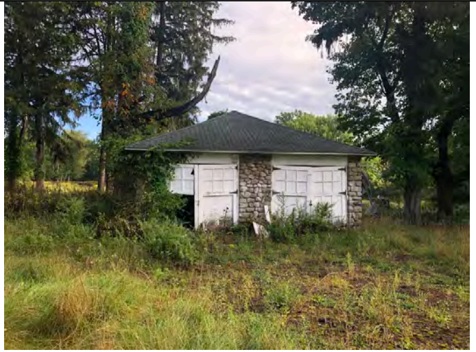
Site Building 2 south exterior
