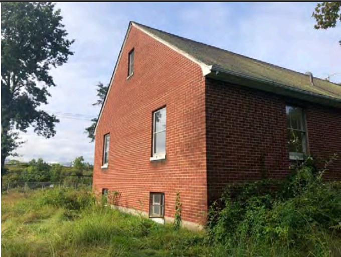
Site Building 1 east exterior
