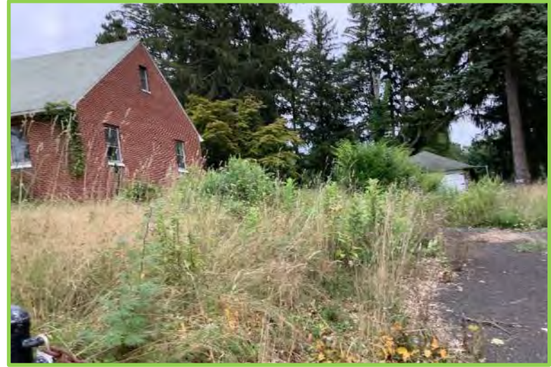
Buildings and disturbed area along Route 17k.
