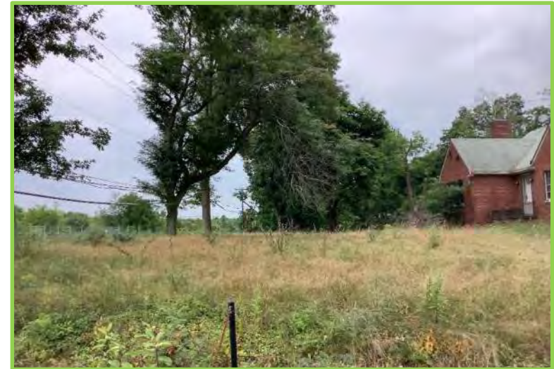
Buildings and disturbed area along Route 17k.
