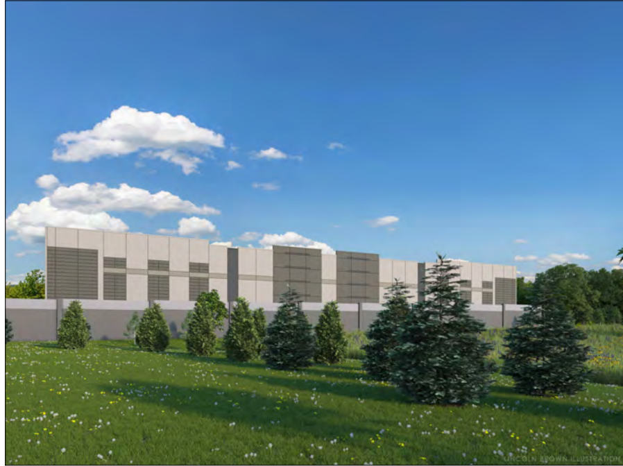
TIME OF PLANTING VIEW FROM 126 ROUTE 17K
