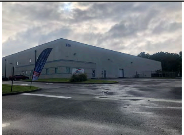
North adjacent property
