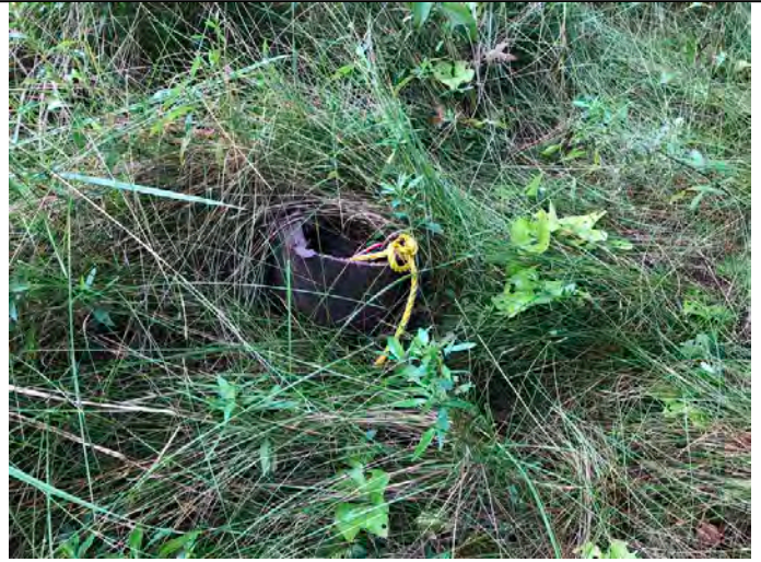
Potable water well northeast of Site Building 1
