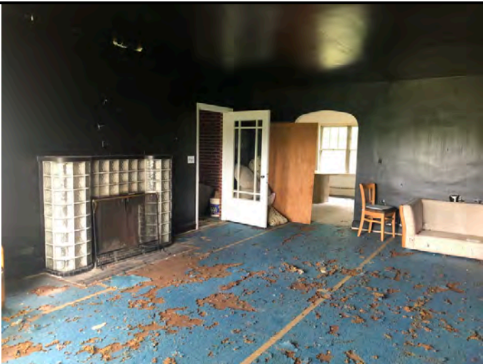
Site Building 1 interior
