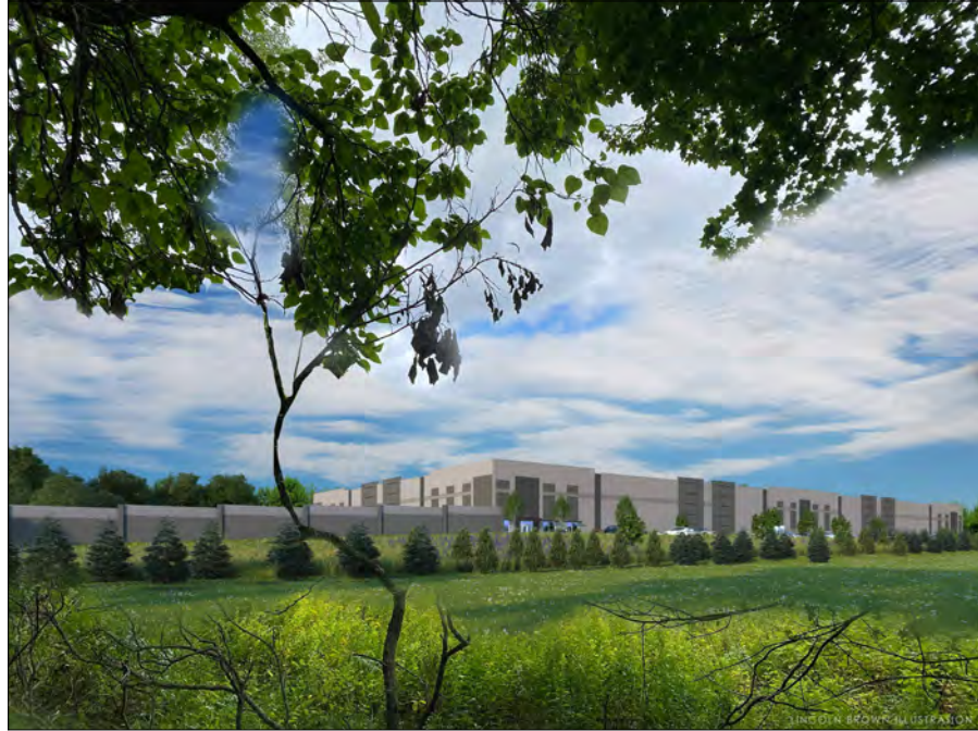
TIME OF PLANTING VIEW FROM 122 ROUTE 17K
