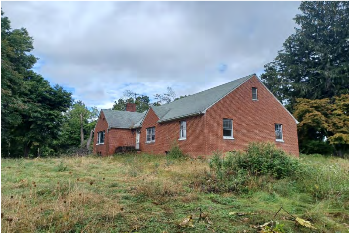
Photo 2: A residential structure is located in the southern portion of the Project APE. The house is vacant. View to the southeast.
