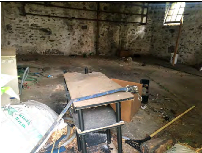
Site Building 2 interior
