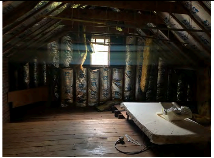
Site Building 1 interior
