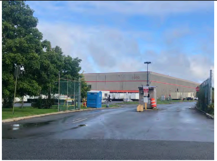
North adjacent property
