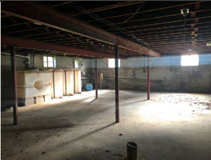
Site Building 1 interior
