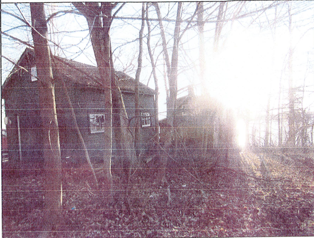
PICTURE # 4 NORTH SIDE OF PROPERTY FROM SUBJECT DRIVEWAY
