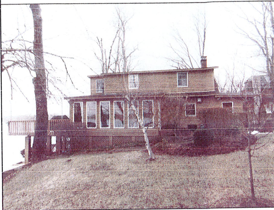
PICTURE # 7 EXISTING LEFT SIDE (SOUTH) OF RESIDENCE
