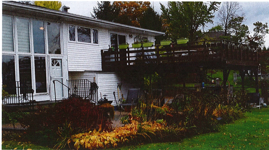
Existing HOUSE & DECK Photo
