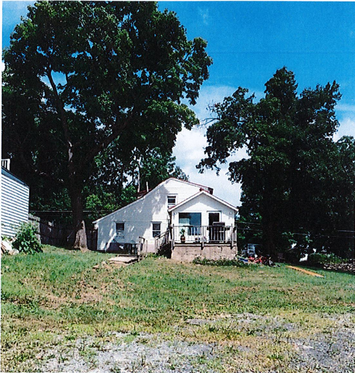
West Side of Property
