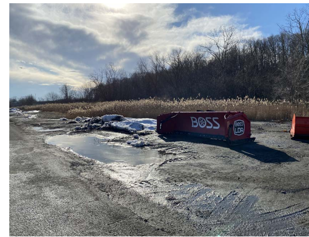
④ EXISTING VIEW OF BEHIND PARKING AREA PROPOSED LOCATION OF GENERATOR & TRANSFORMER
