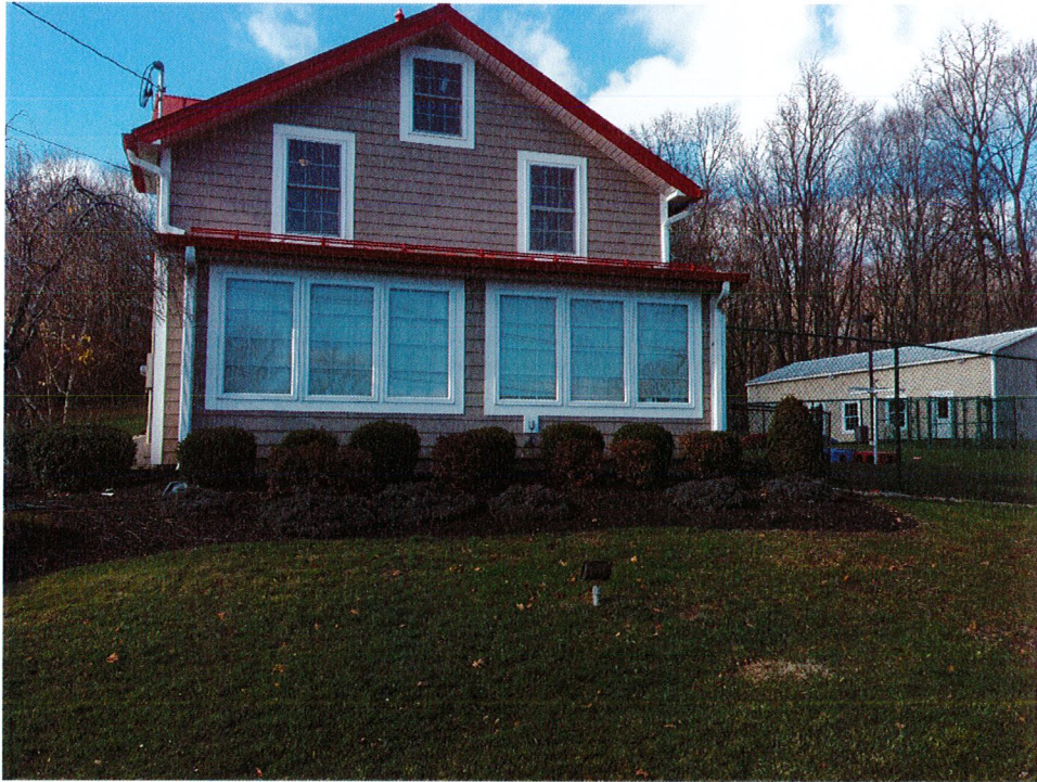
Front view of existing structure (East)
