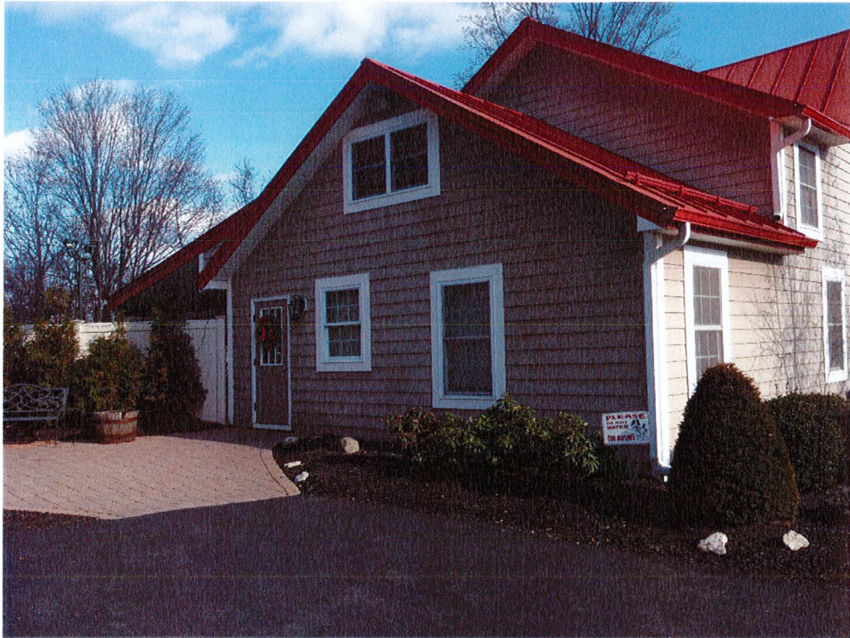
Rear view of existing structure (West)
