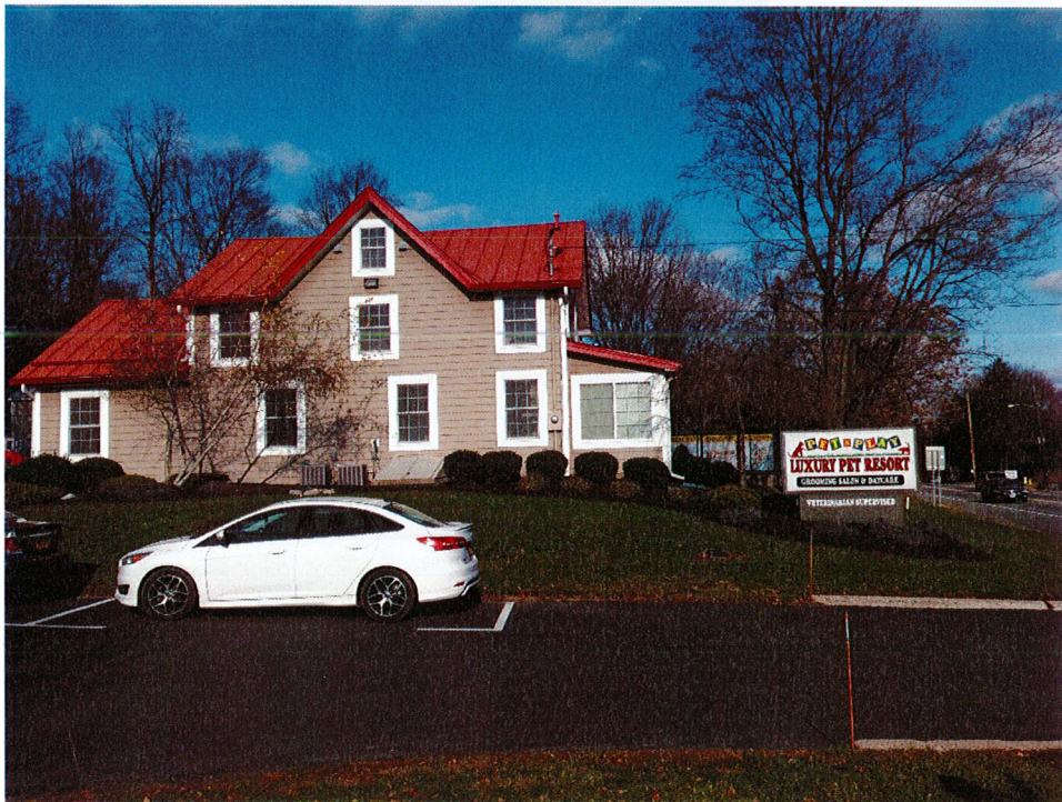
Side view of existing structure (South)
