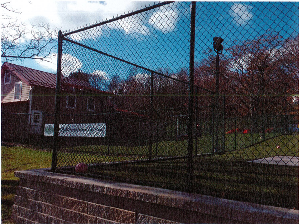
Side view of existing structure (North)
