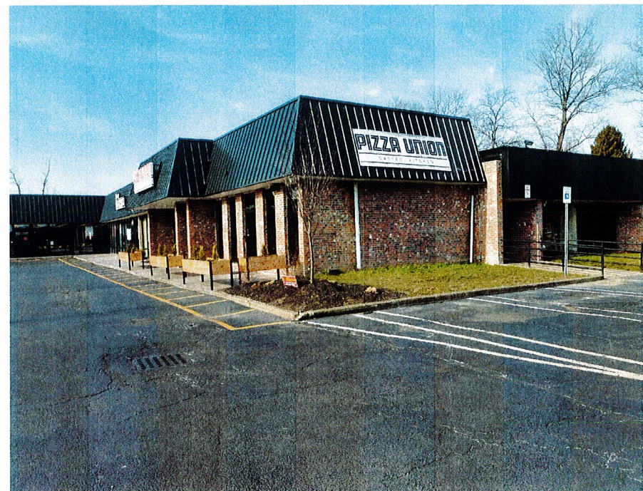
3 EXISTING SITE PHOTO
