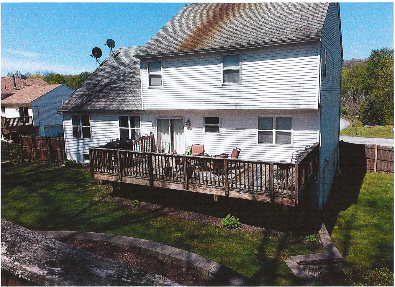
REAR NEIGHBOR - 20 RAMBLEWOOD DRIVE S/B/L 117-4-11
