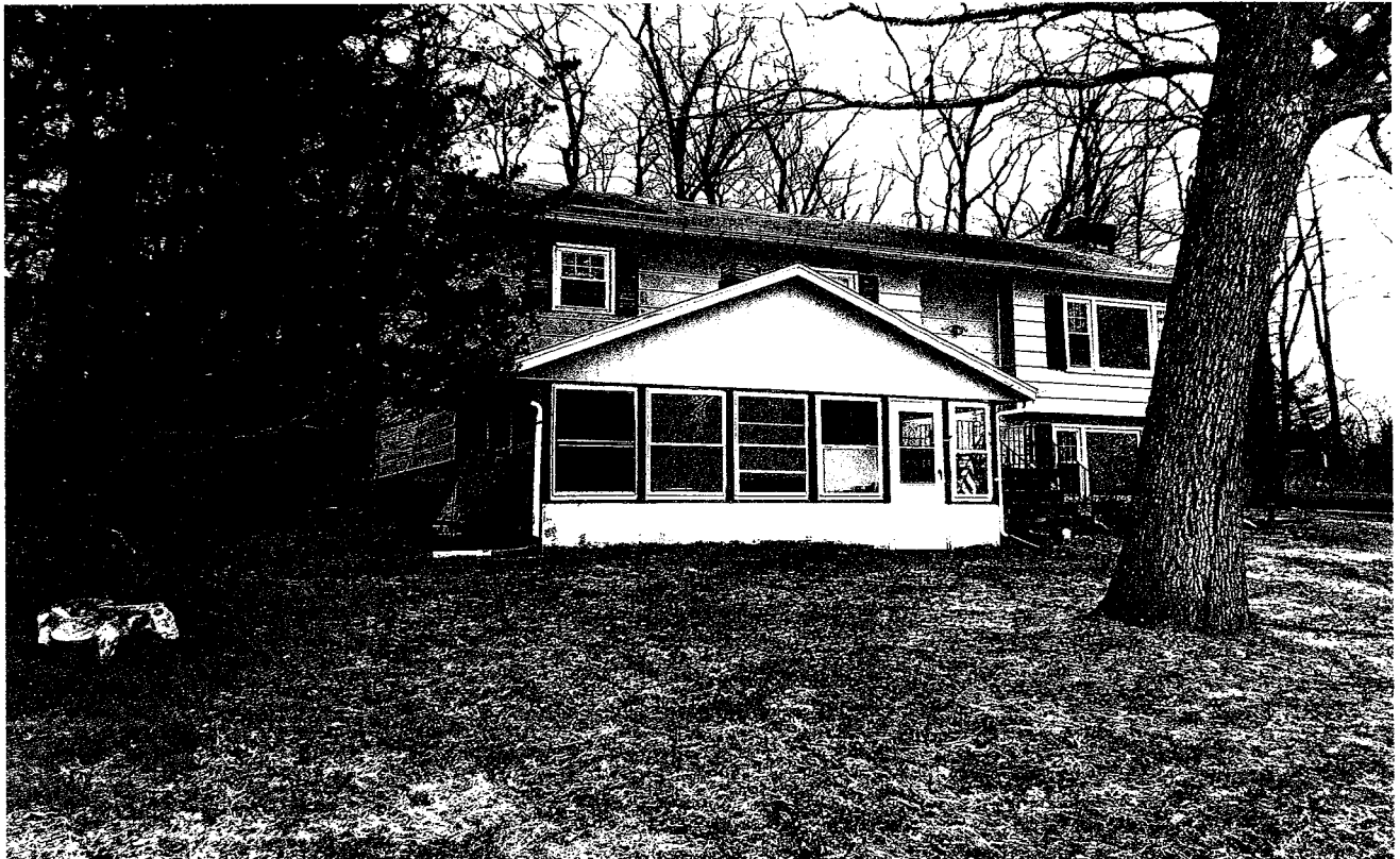
Taken from NORTH WEST corner looking south
