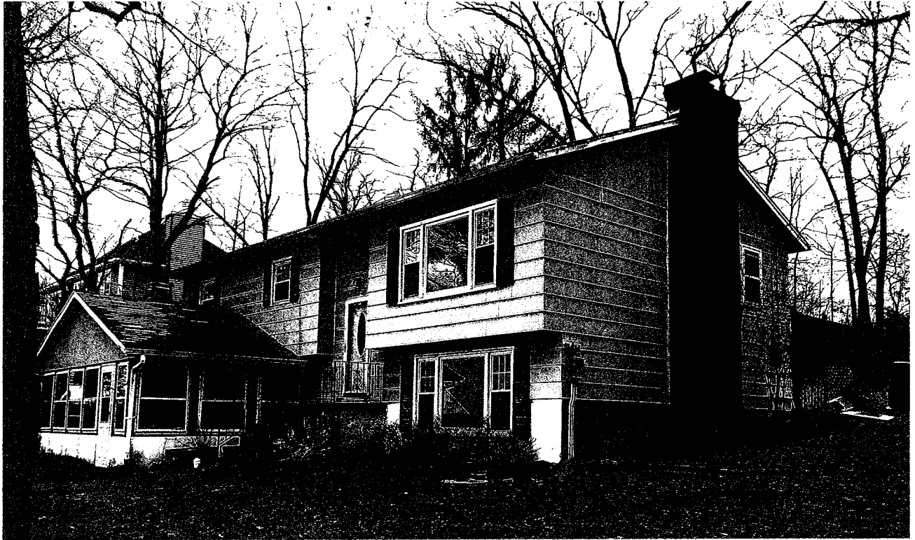
Taken from SOUTH WEST corner looking north
