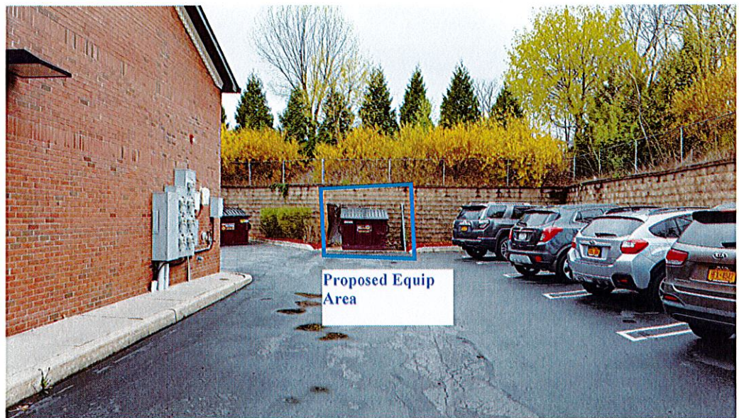
View of existing dumpster area and proposed equipment compound area (SW area of site).
