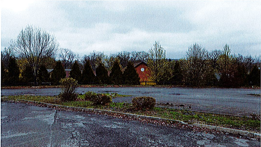
Existing View of rear of existing building from cinema property (looking N-NE).
