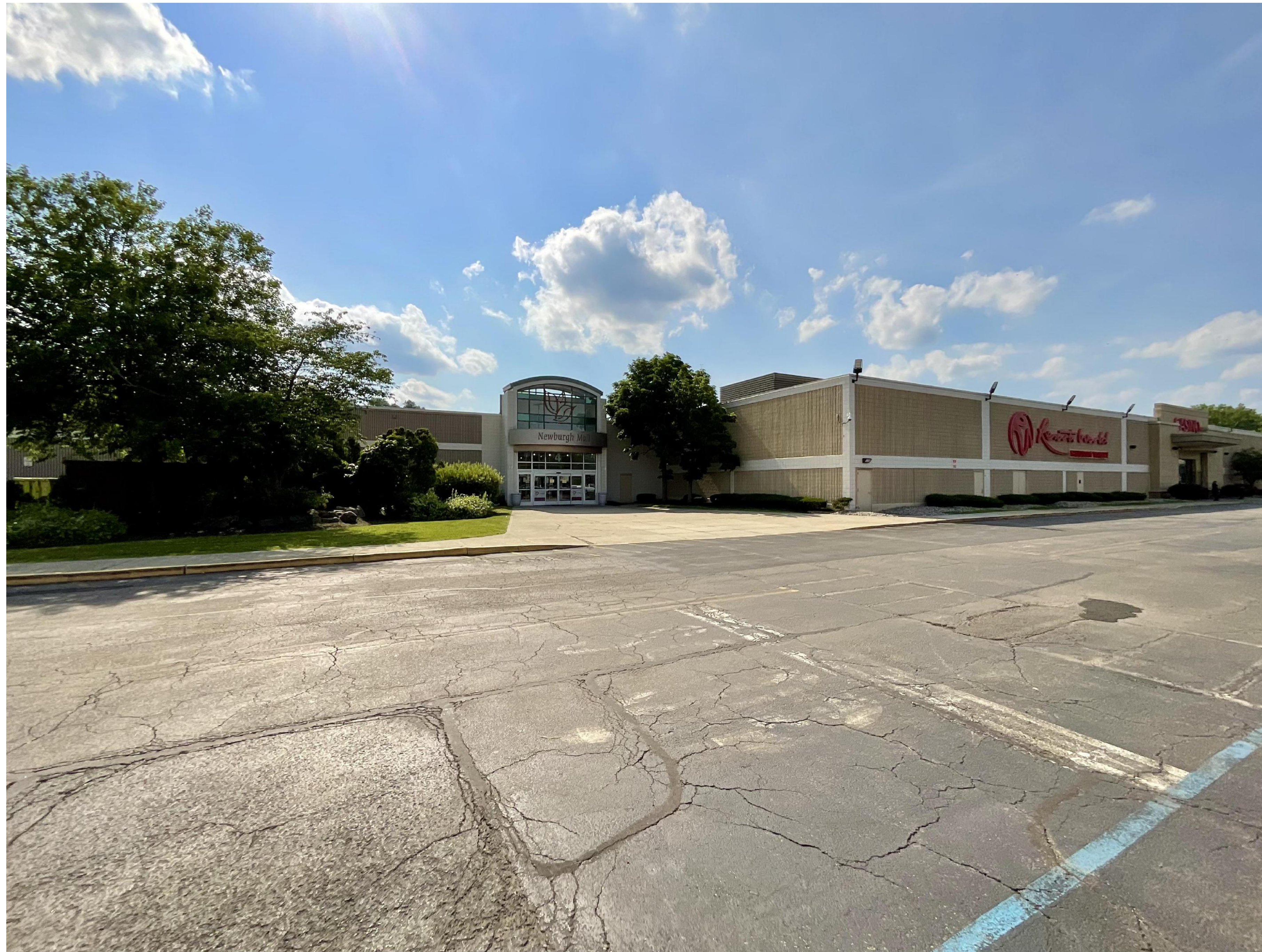
① EXISTING MALL IMAGE FROM EAST 1" = 1'-0"
