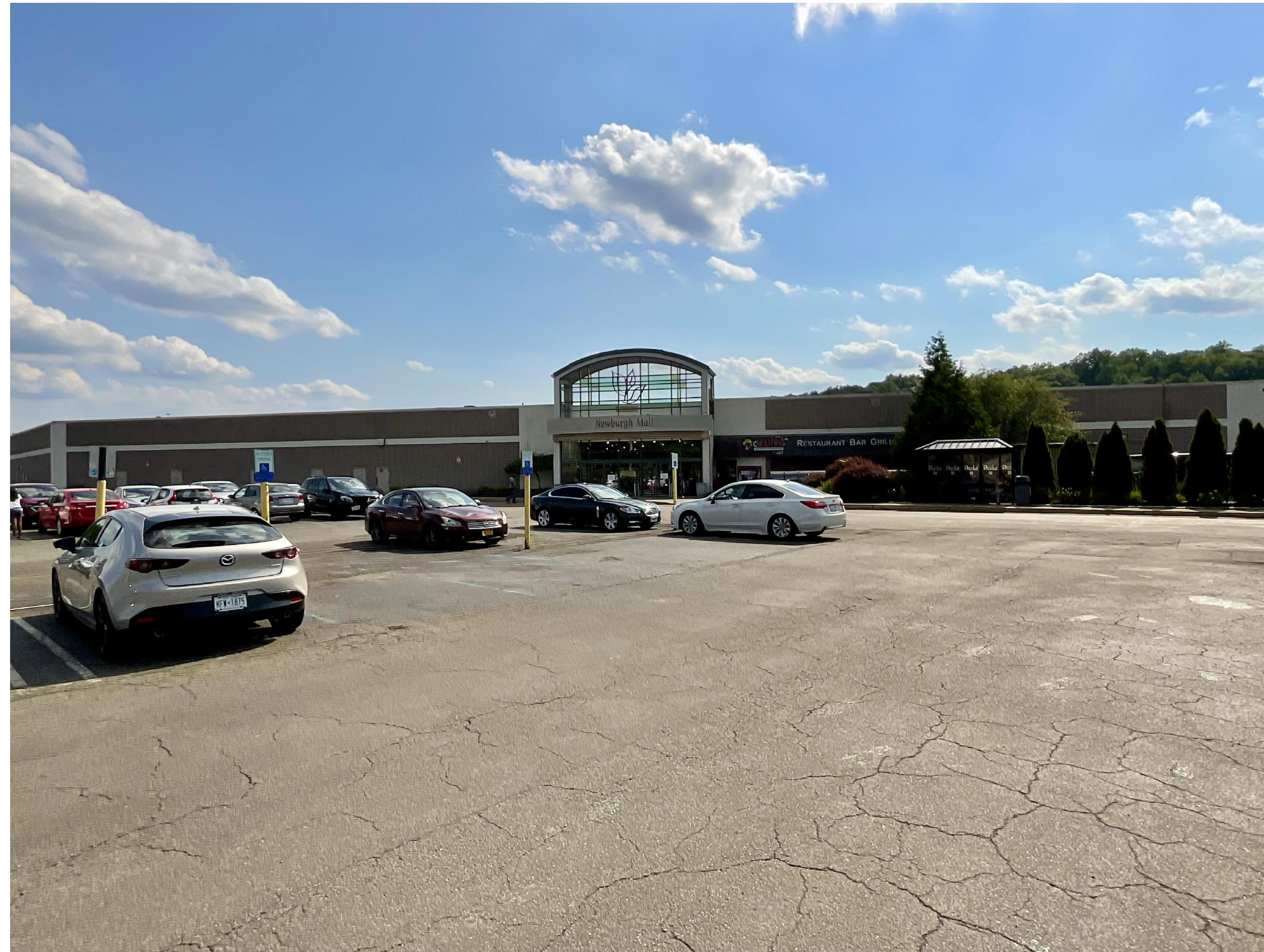
1 EXISTING MALL IMAGE FROM EAST 1" = 1'-0"
