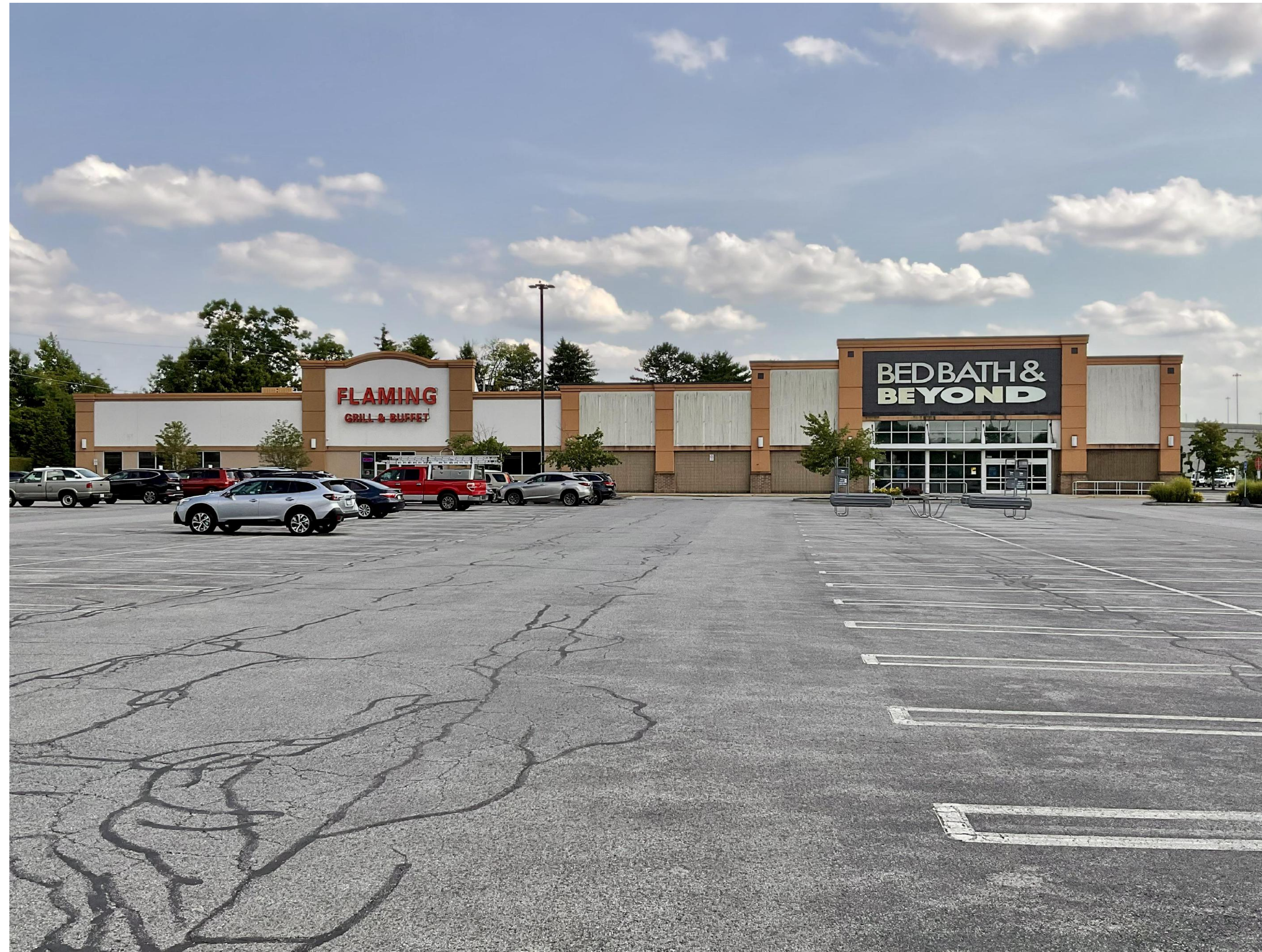
1 EXISTING OUTER PARCEL IMAGE FROM SOUTH WEST 1" = 1'-0"
