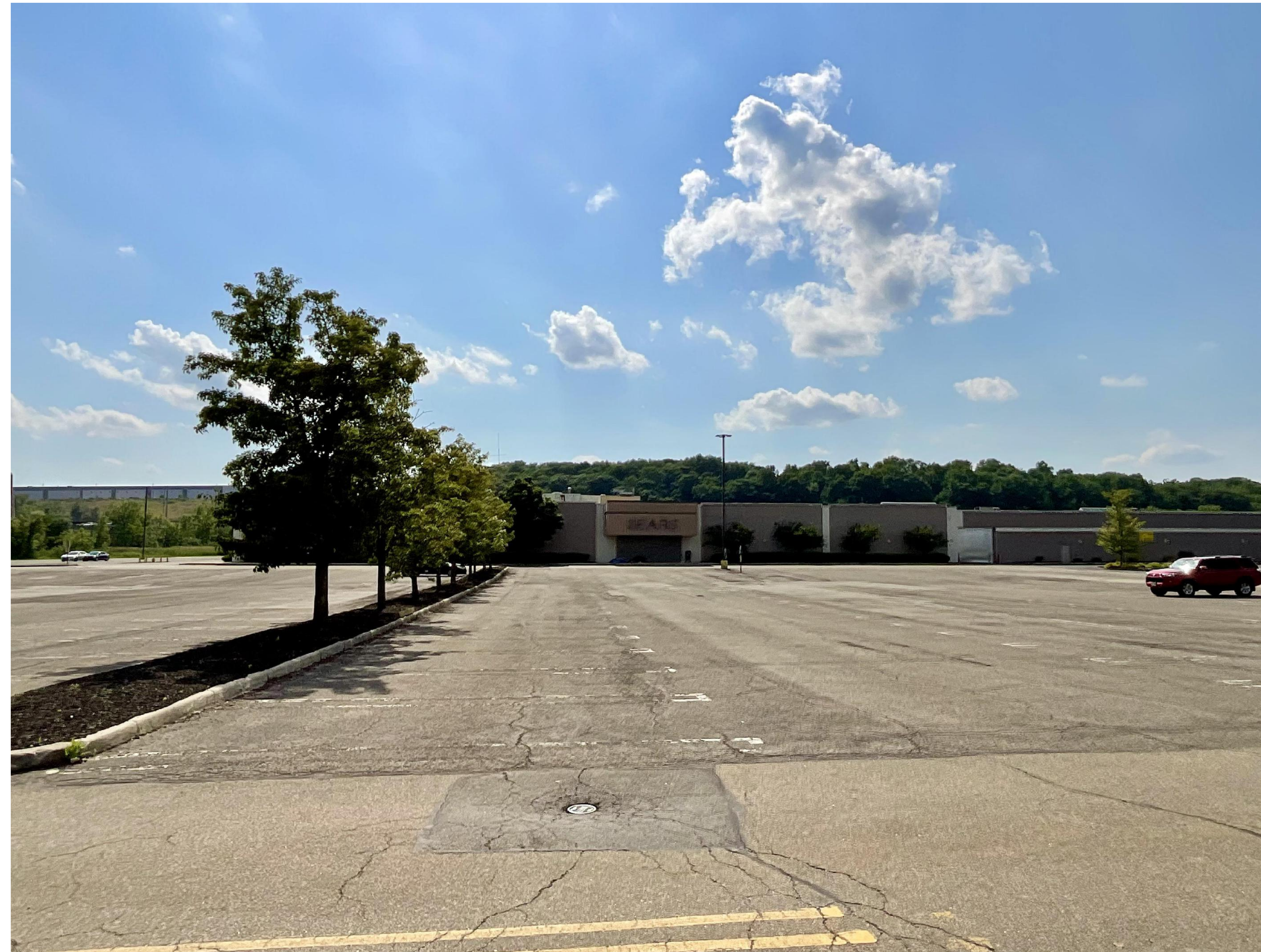
① EXISTING MALL IMAGE FROM EAST 1" = 1'-0"
