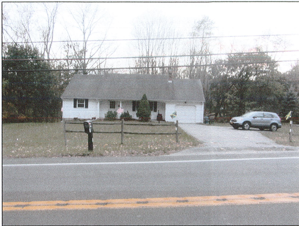
PICTURE # 1 PROPERTY FRONTAGE ALONG NYS ROUTE 300 (NORTH ELEVATION)
