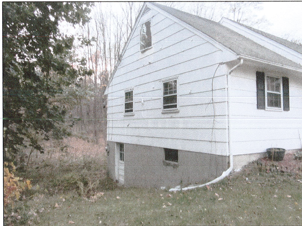
PICTURE # 4 LEFT SIDE ELEVATION EAST ELEVATION
