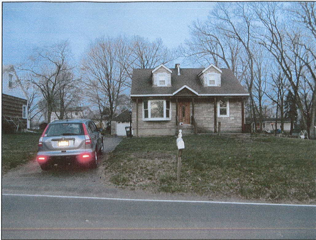
PICTURE # 1 FRONT (WEST) SIDE ELEVATION
