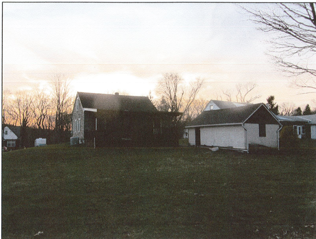
PICTURE # 4 REAR (EAST) SIDE ELEVATION
