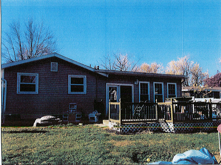
PHOTO OF NEW ADDITION
