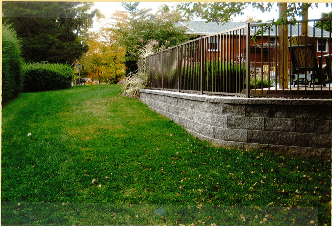
REAR SOUTH CORNER OF PROPERTY (47-1-8.3) FACING WEST.
