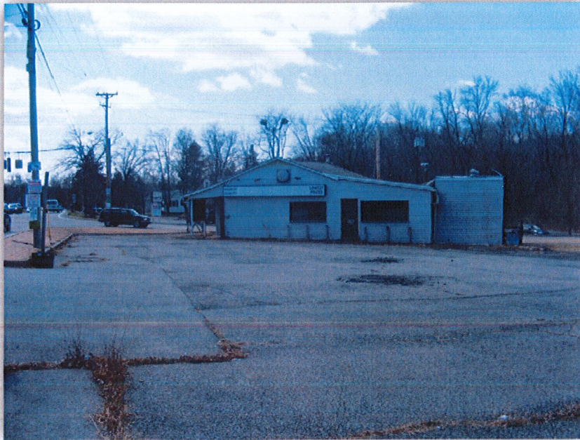
North Elevation Photographed on 04.09.2014
