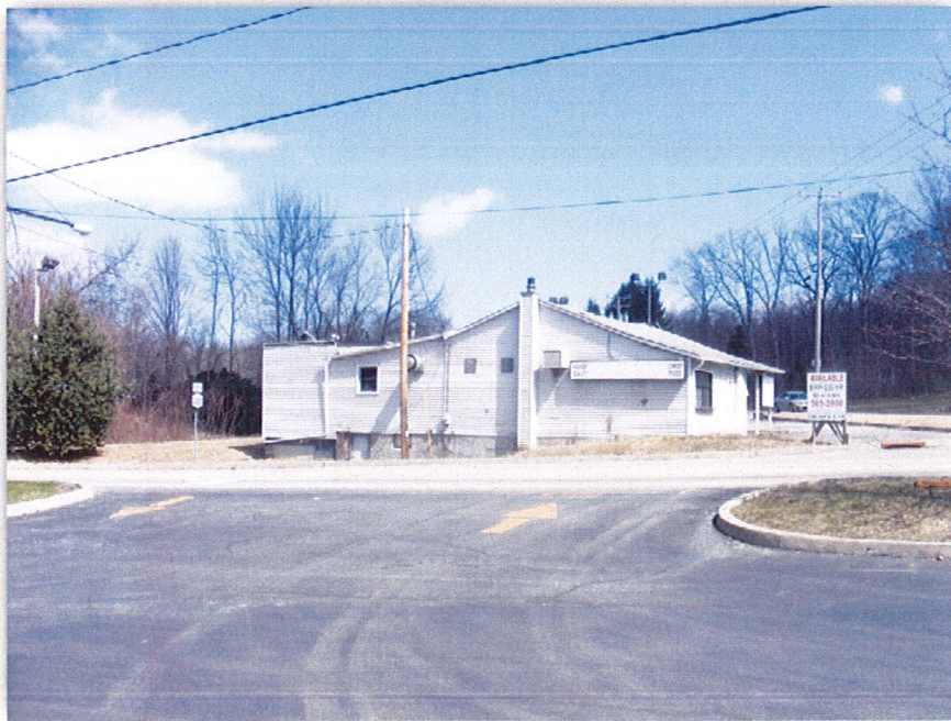
South Elevation on Route 32 Photographed on 04.09.2014
