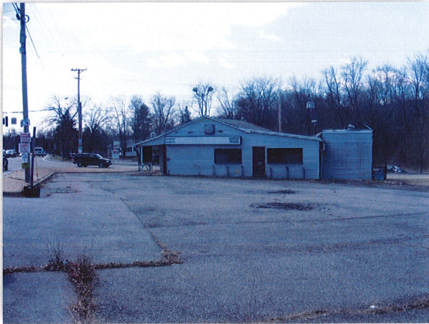
North Elevation Photographed on 04.09.2014
