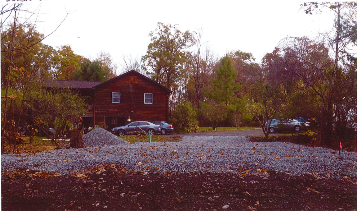
Back of building area toward front of property (house)
