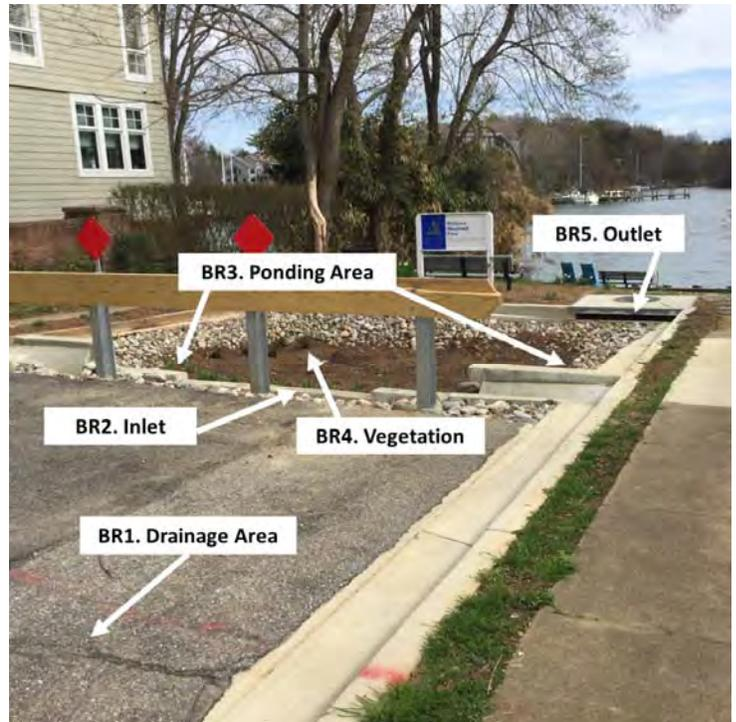
**Figure 2.7.1.** Key Areas for Level 1 Inspection of Bioretention
