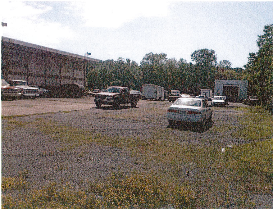
Looking southwesterly towards the existing building.
