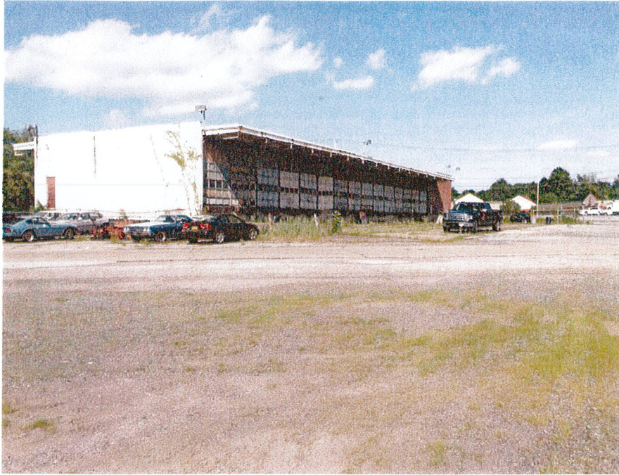
Looking northeasterly towards the existing building.
