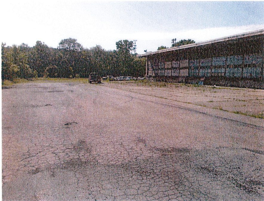
Looking northwesterly towards the existing building.
