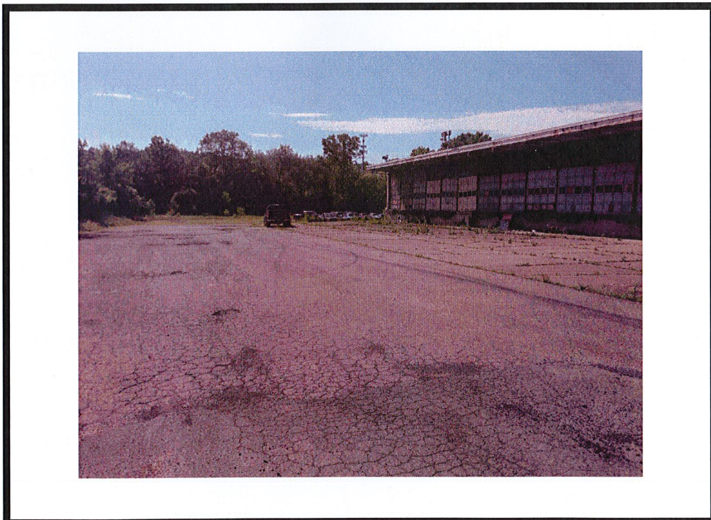
Looking northwesterly towards the existing building.
