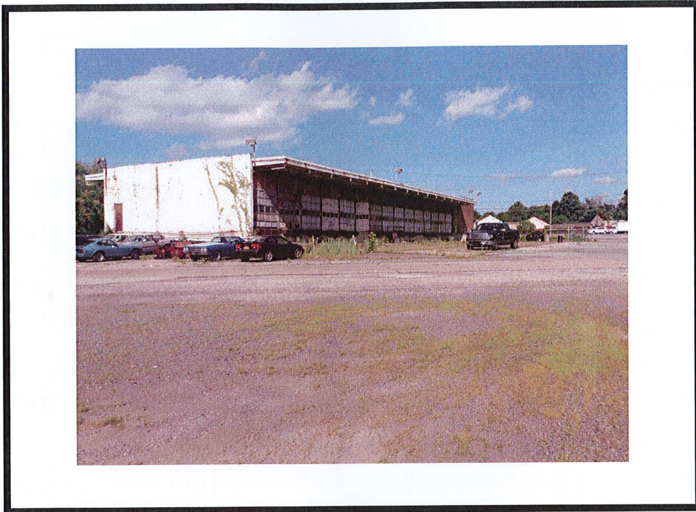
Looking northeasterly towards the existing building.
