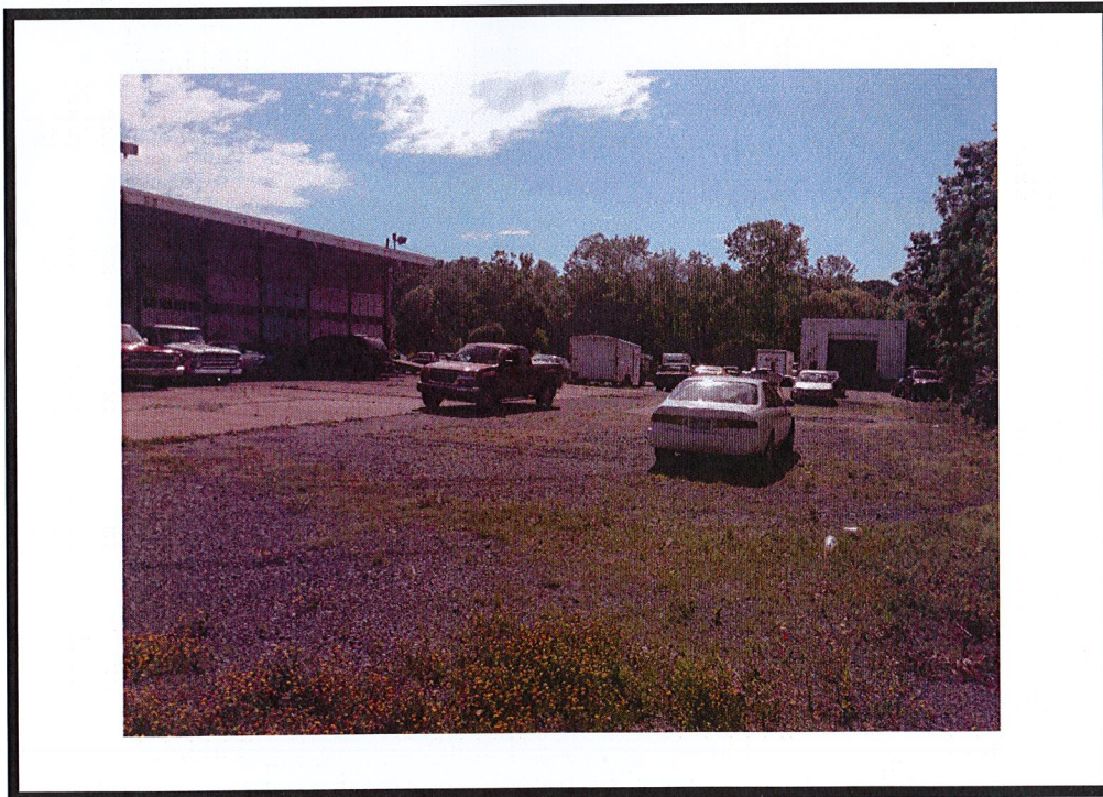
Looking southwesterly towards the existing building.
