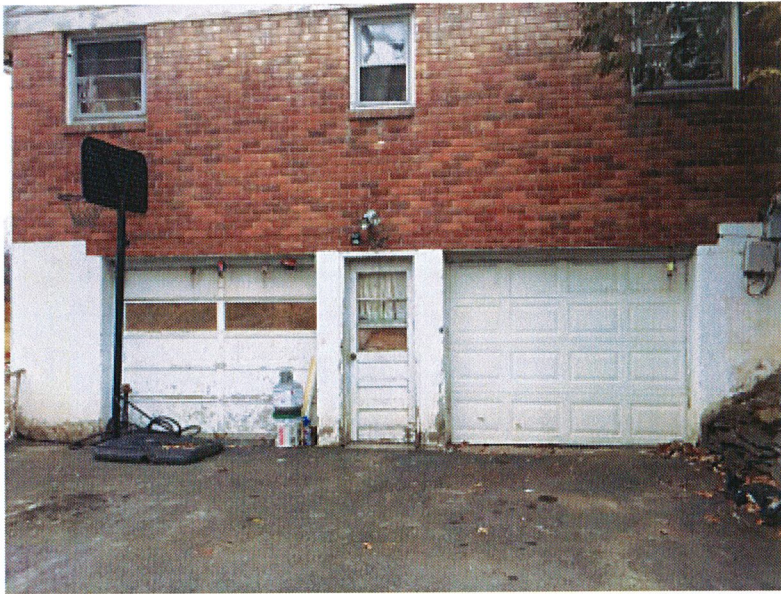
VIEW OF THE ATTACHED GARAGE
