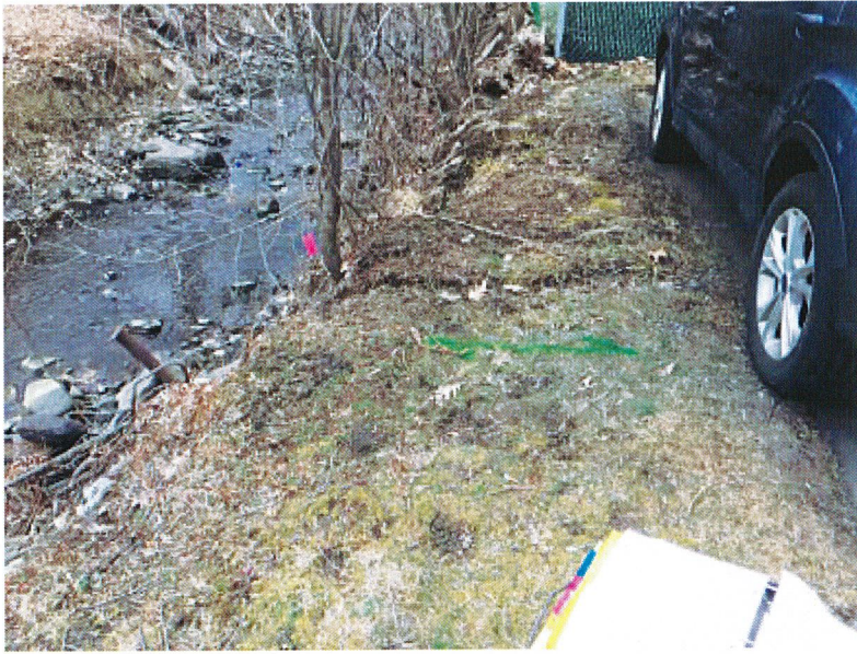
VIEW OF THE STORMWATER DISCHARGE INTO THE CREEK
