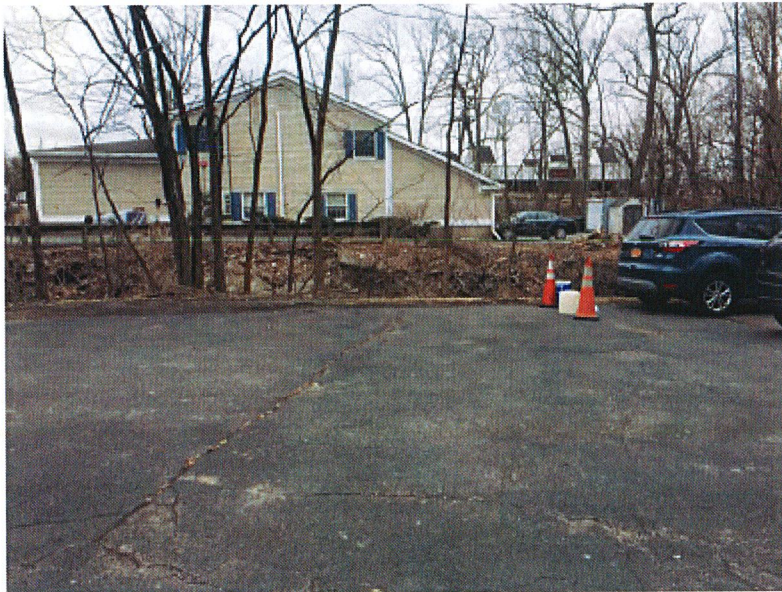
VIEW OF THE ASPHALT PAVED DRIVEWAY
