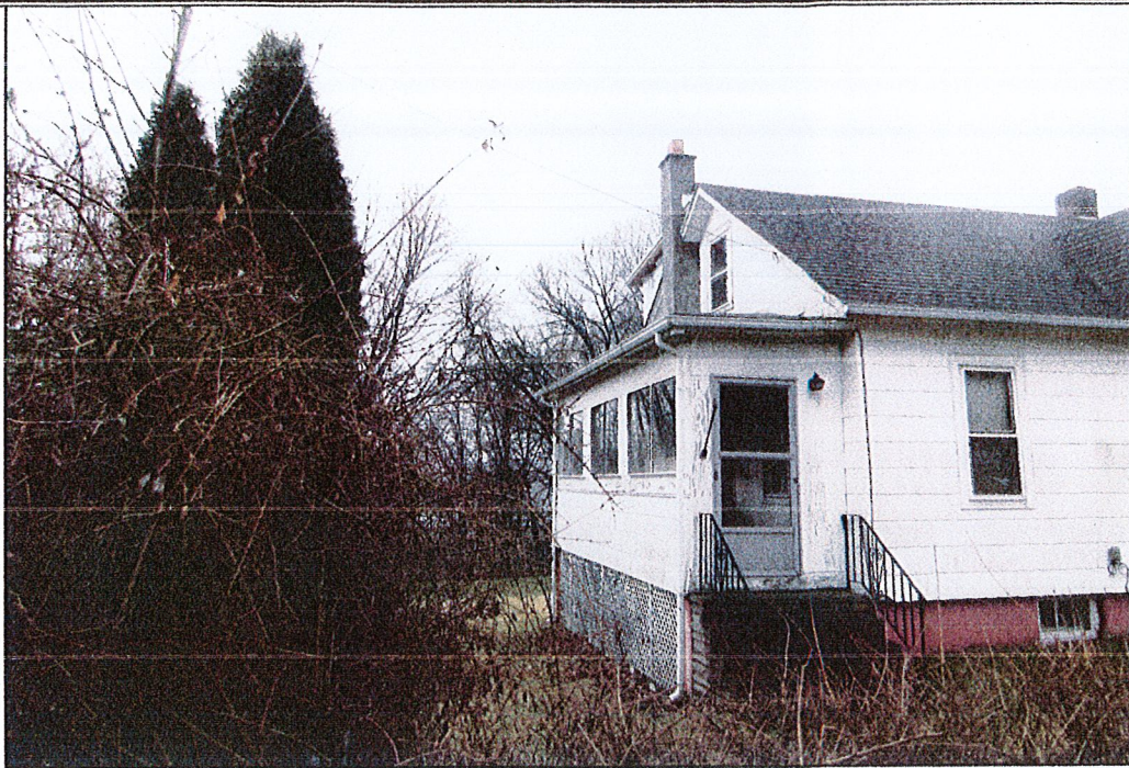
PICTURE # 3 LEFT (EAST) SIDE OF PROPERTY FROM TERRY AVENUE
