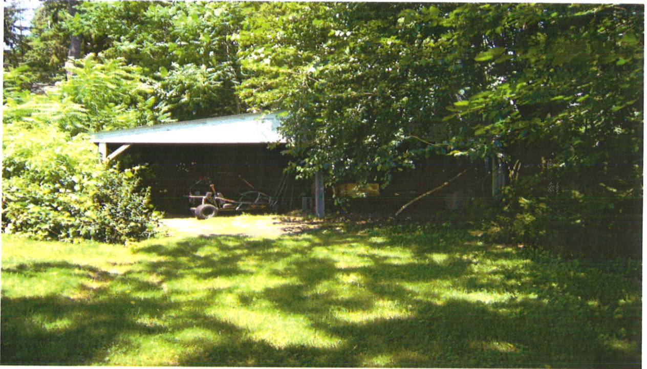
3. View of pole barn looking northwest.
