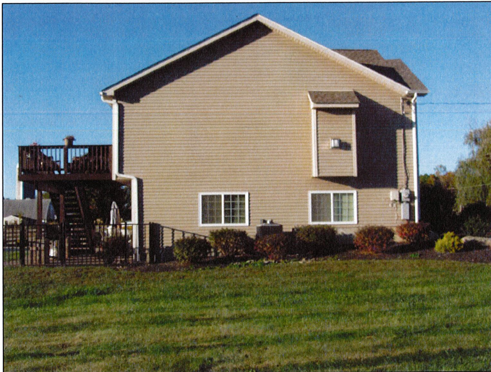
PICTURE # 4 LEFT (SOUTH) SIDE ELEVATION
