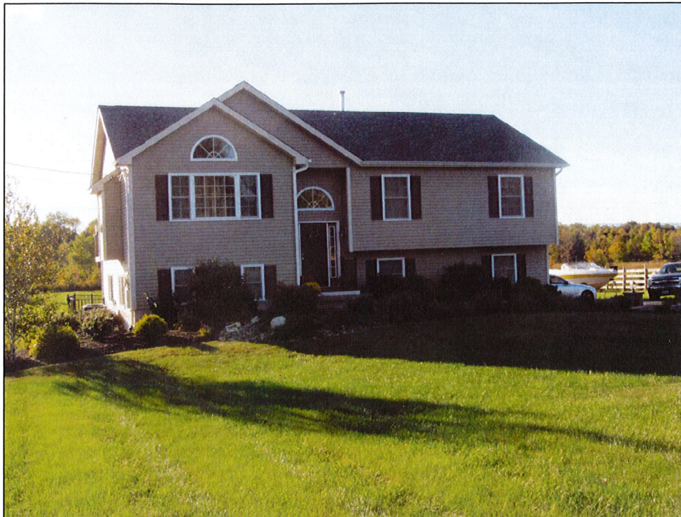
PICTURE # 1 FRONT (EAST) SIDE ELEVATION
