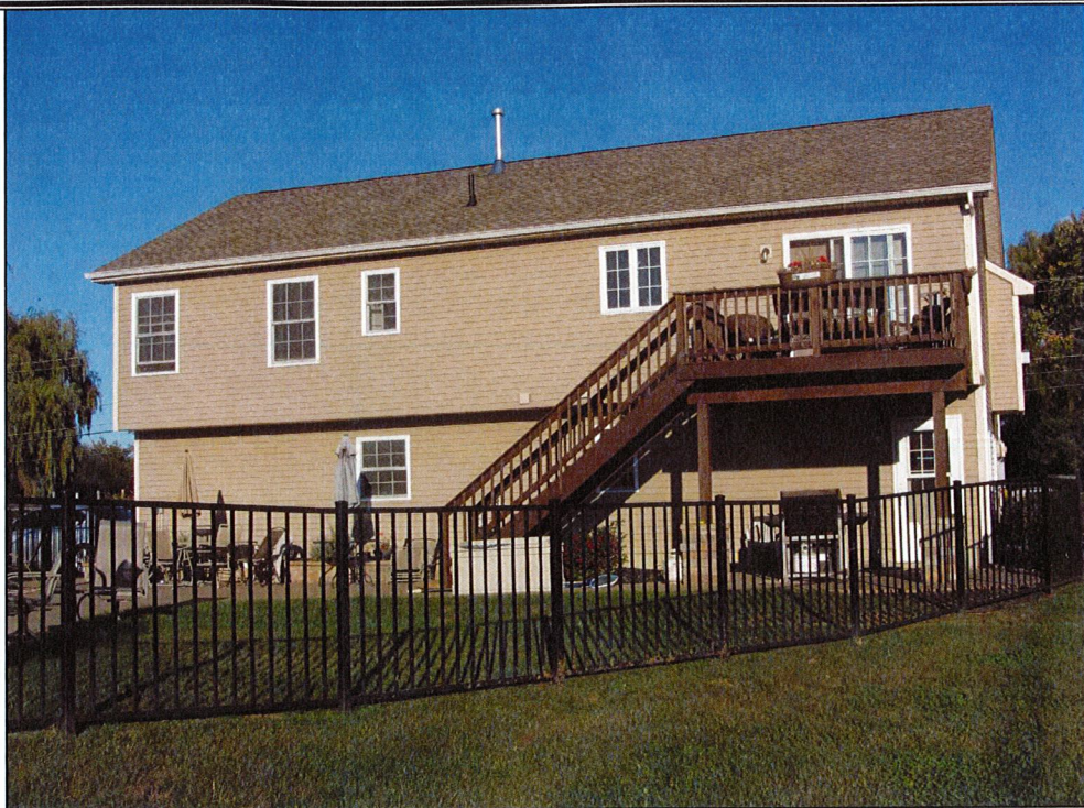
PICTURE # 3 REAR (WEST) SIDE ELEVATION
