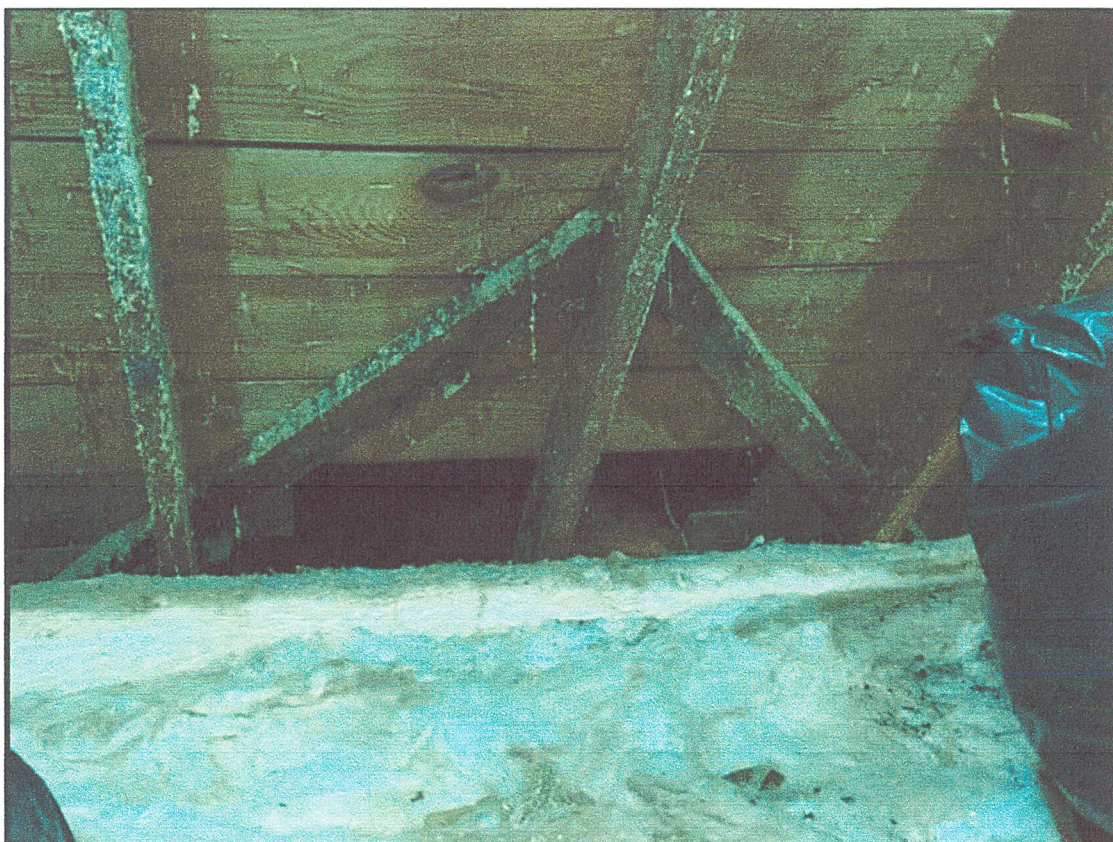
Shared insulated attic space over enclosed porch
