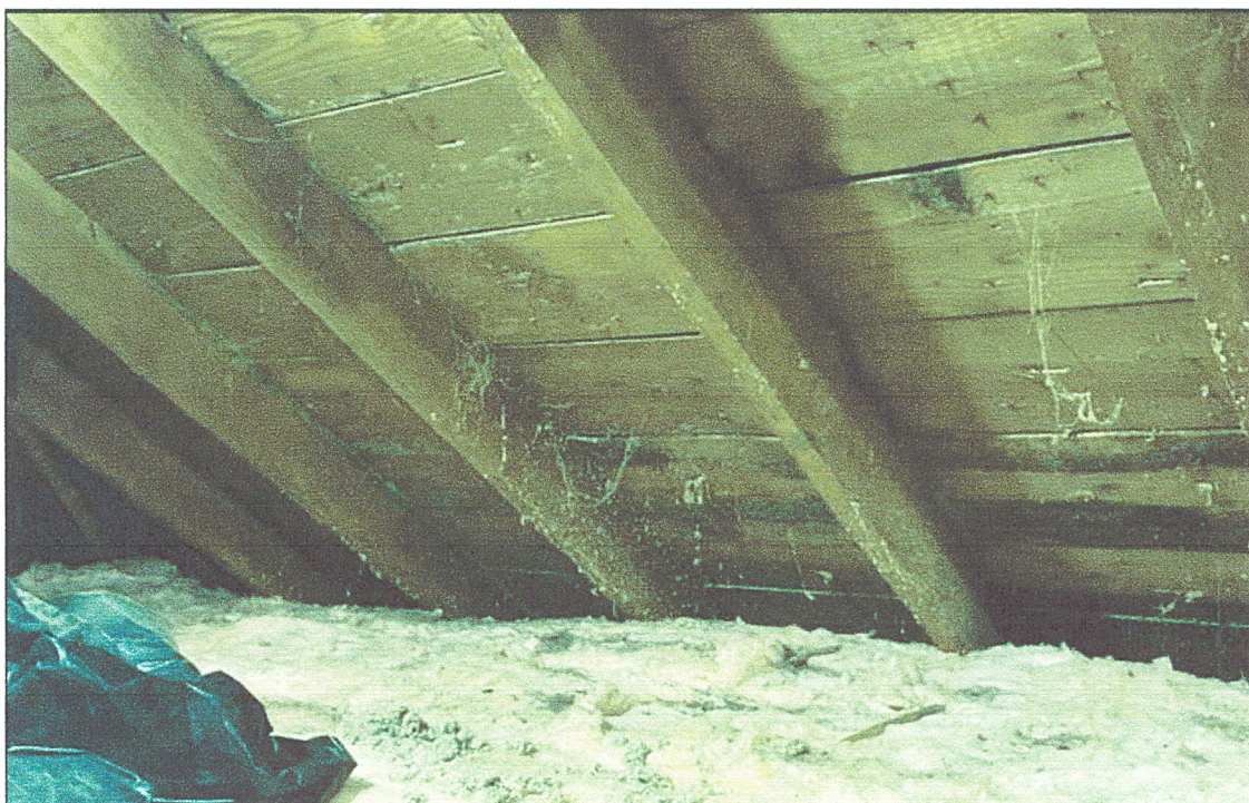
No attic space over non-enclosed stoop/covered porch
