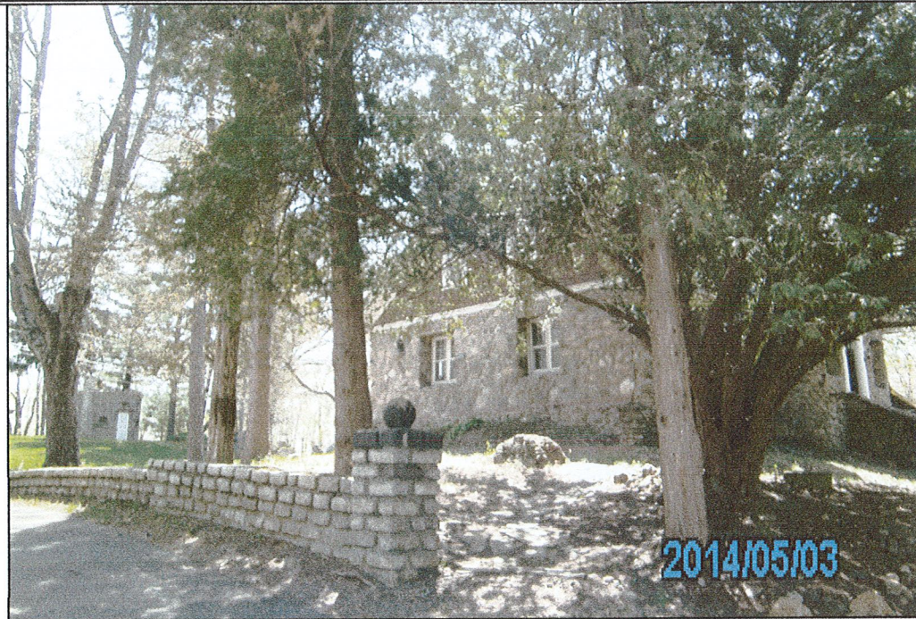
PICTURE # 3 PARTIAL FROM FRONT AND SIDE FROM EAST VIEW ROAD
