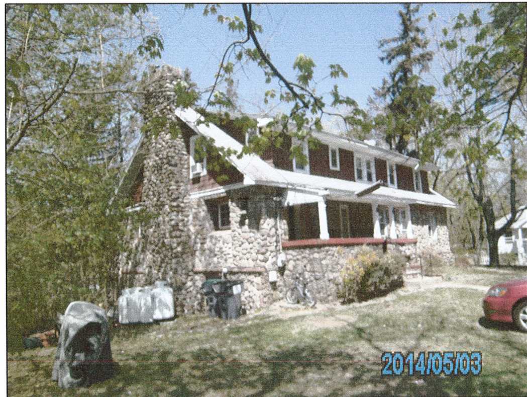
PICTURE # 6 REAR AND SOUTH SIDE FROM CHEVY LANE
