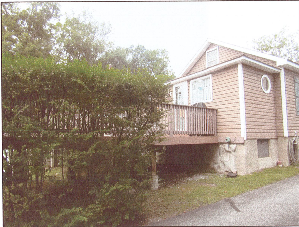
PICTURE # 4 SOUTHWEST SIDE OF PROPERTY FROM SUBJECT DRIVEWAY
