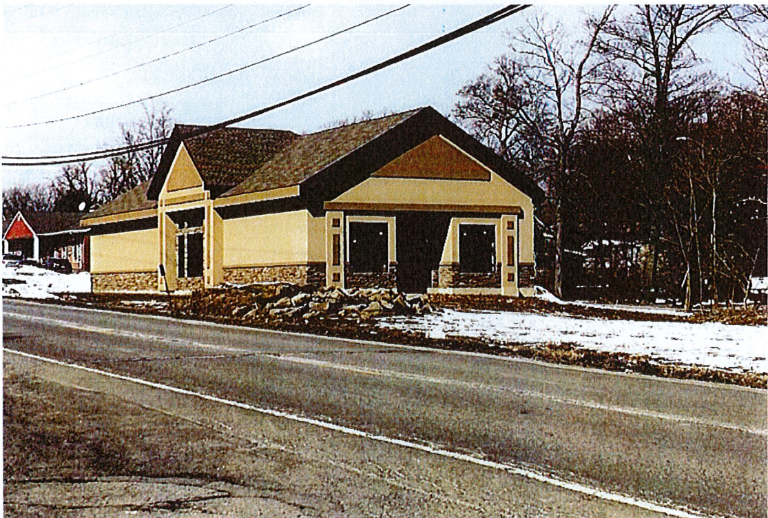
View West from NYS Route 52
