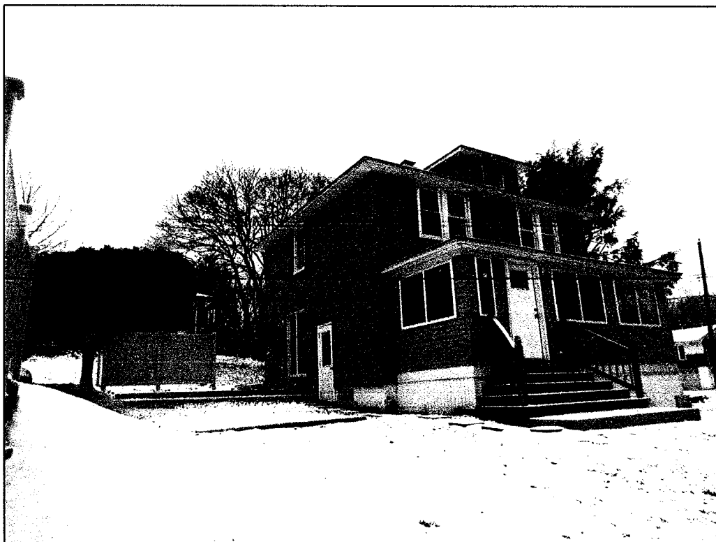
PICTURE # 2 PARTIAL FRONT/SIDE ELEVATION HY VUE DRIVE
