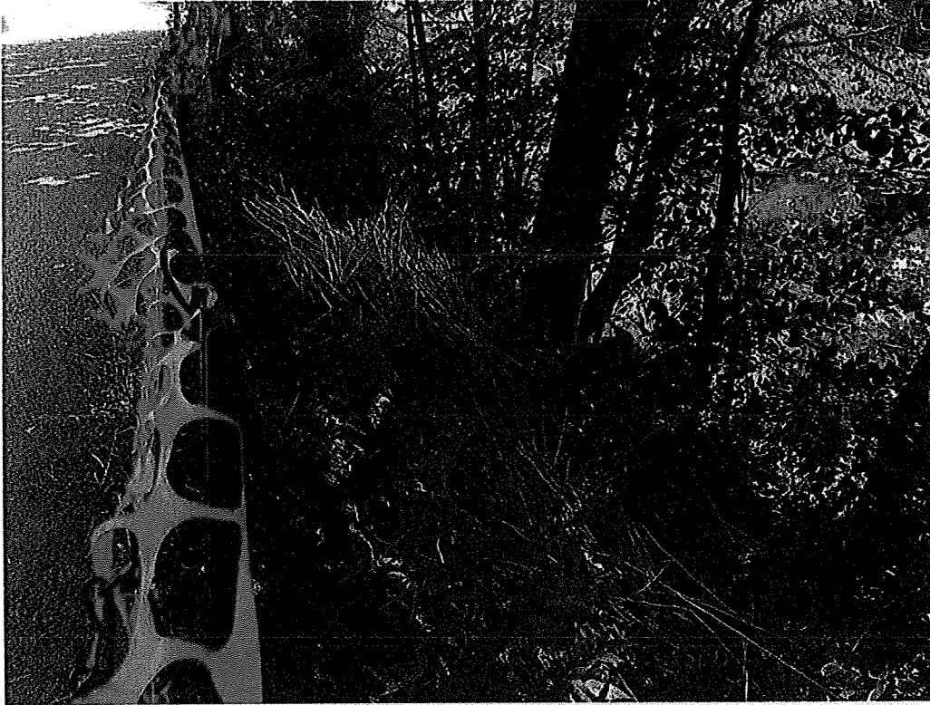
EMBANKMENT SLOPE DOWN TO THE CREEK
