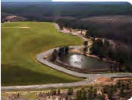
Baldwin County Landfill, GA
