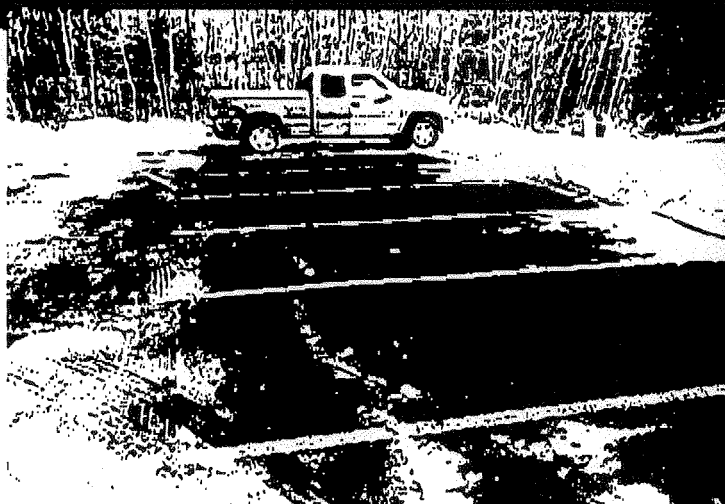
Figure 3. Comparison of dense-mix asphalt (left) and porous asphalt (right) on the same day, one hour after blowing.
