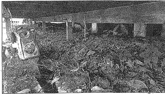
PHOTO OF EXISTING CONDITIONS
