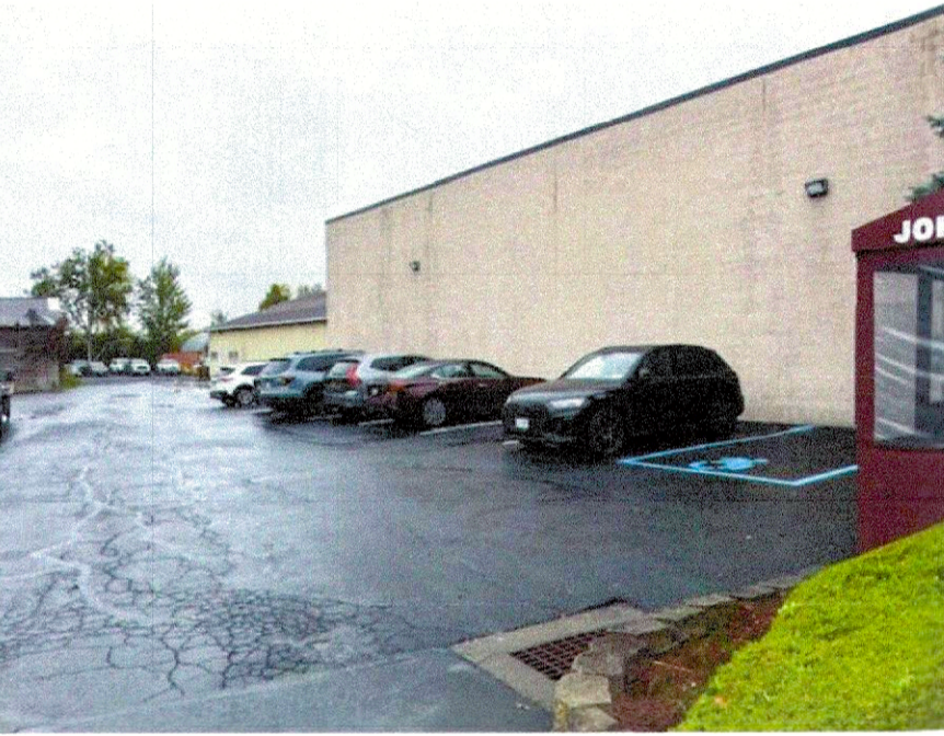
7 PARKING SPACES EXISTING EXTERIOR LIGHTS
