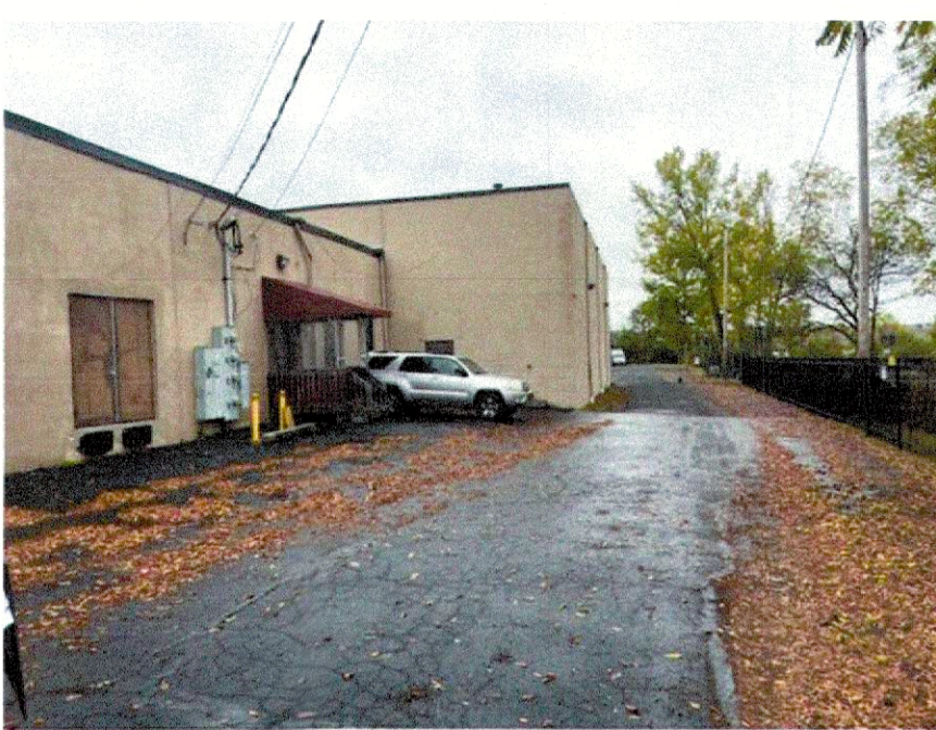
EXISTING EXTERIOR LIGHT
