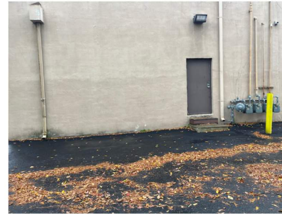
EXISTING EXTERIOR LIGHT
