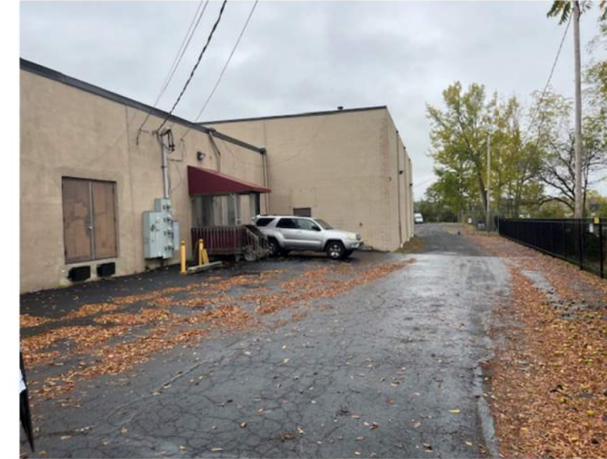
EXISTING EXTERIOR LIGHT
