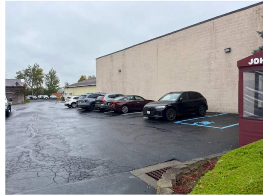
7 PARKING SPACES EXISTING EXTERIOR LIGHTS
