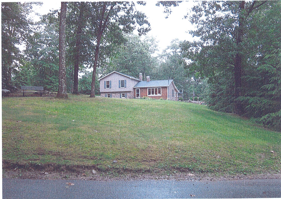
Front Carpenter's House from Decker Road
