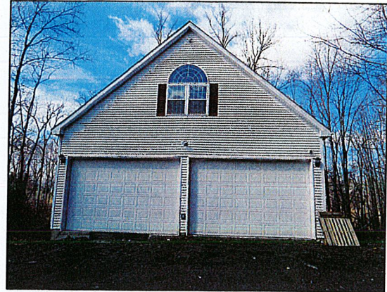
PHOTO OF EXISTING STRUCTURE
