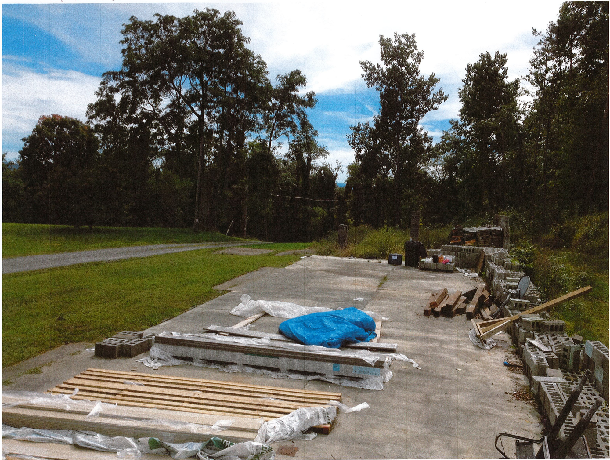
7 MANZO RD LOOKING SOUTH OVER EXISTING FOUNDATION + SLAB
