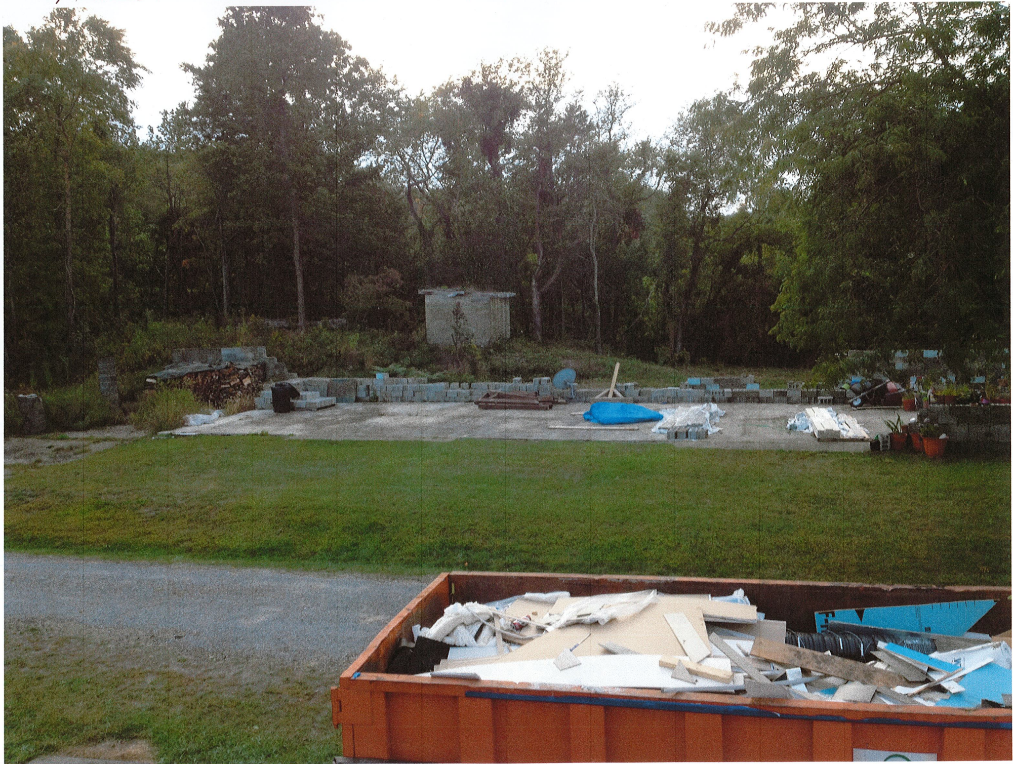
7 MANZO RD LOOKING WEST AT PROPOSED GARAGE SITE
