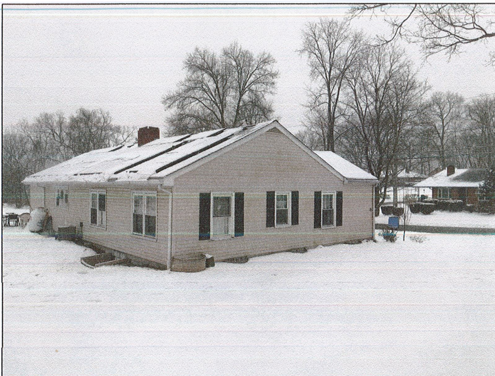
PICTURE # 2 PARTIAL SIDE/REAR YARD
