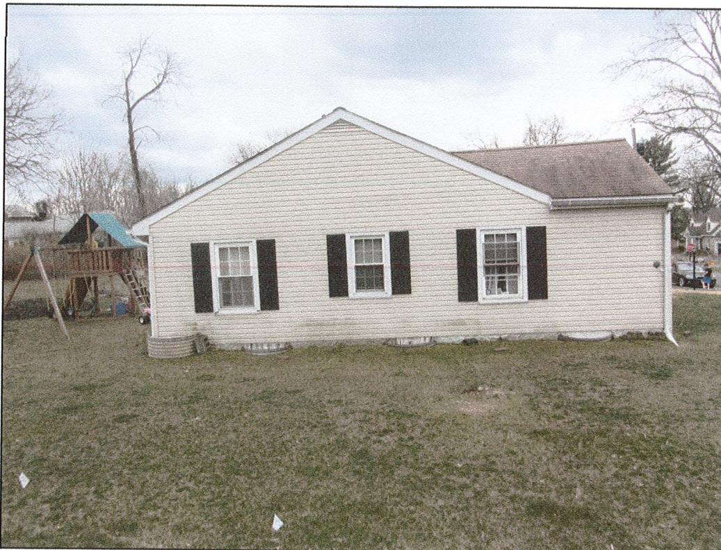
PICTURE # 6 NORTH ELEVATION CHEVY LANE
