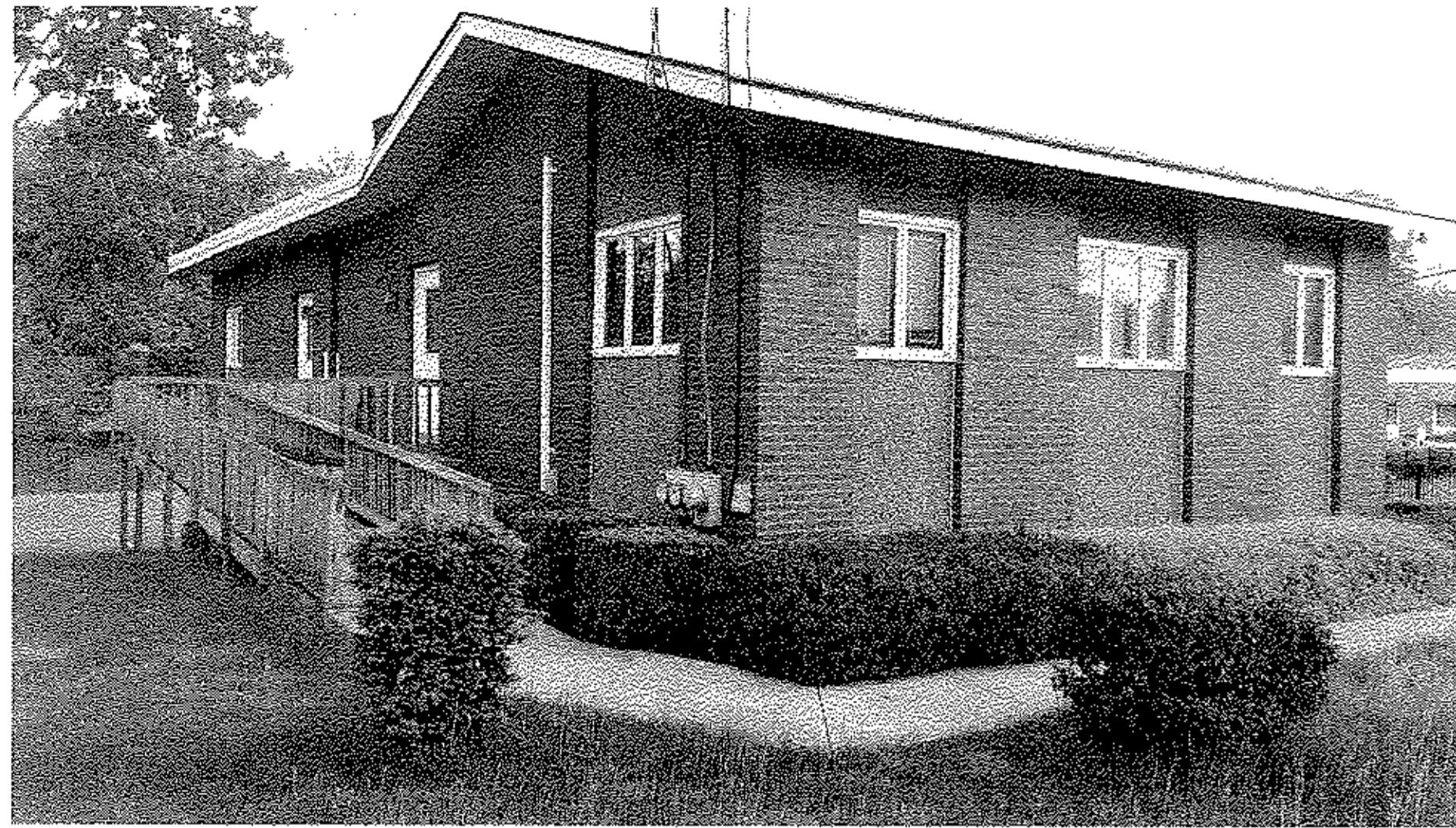
1 SITE PHOTO - SOUTH WEST SIDE EX-2
