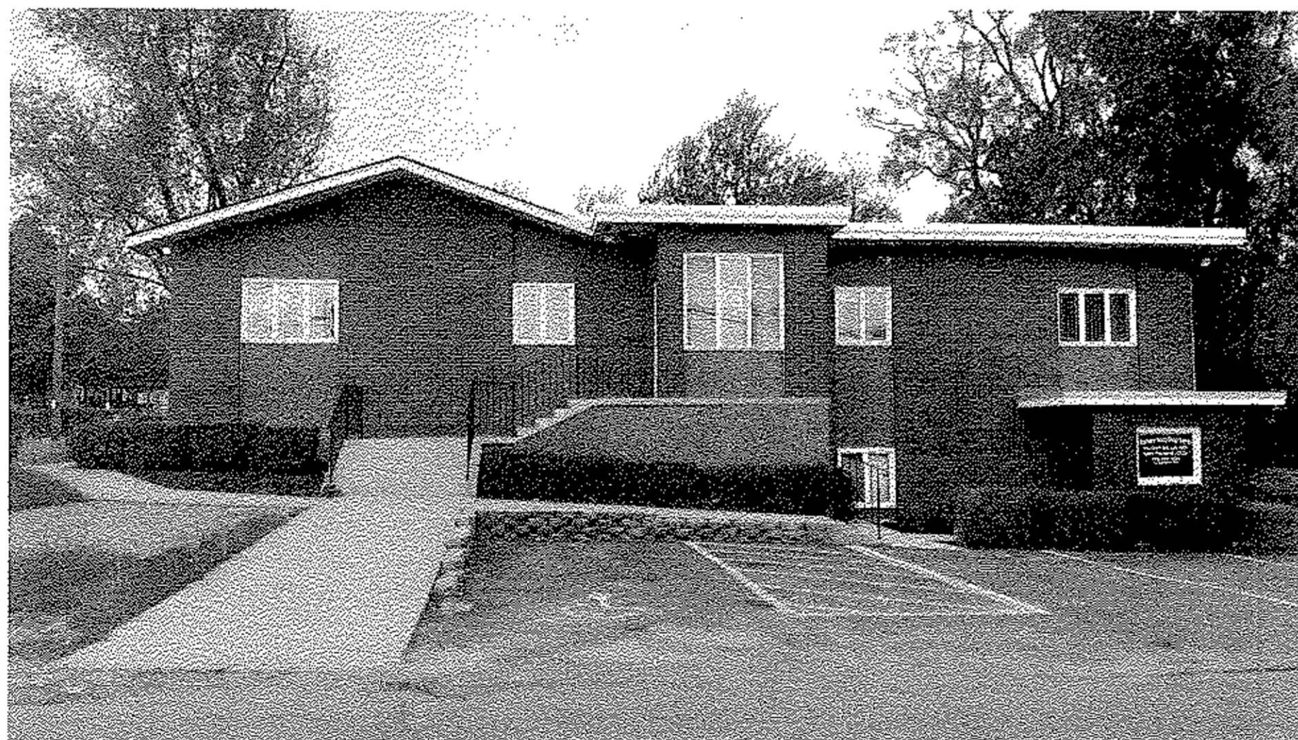
4 SITE PHOTO - EAST SIDE EX-2
