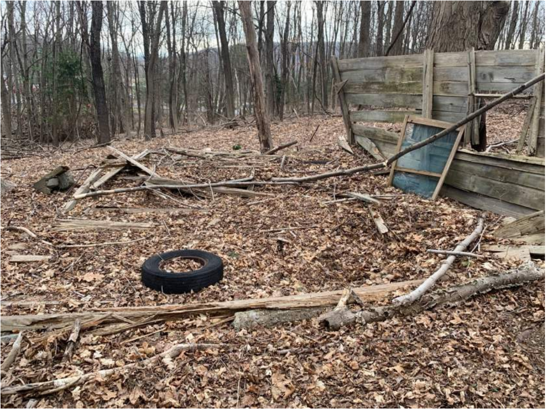
Remains of Shed or garage structure southeast of house
