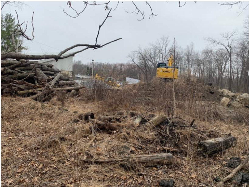
CHG&E Materials Storage area near southwest corner of SP
