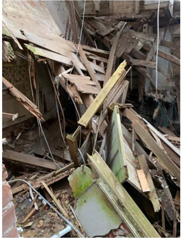
Collapsed floor area inside house from south window
