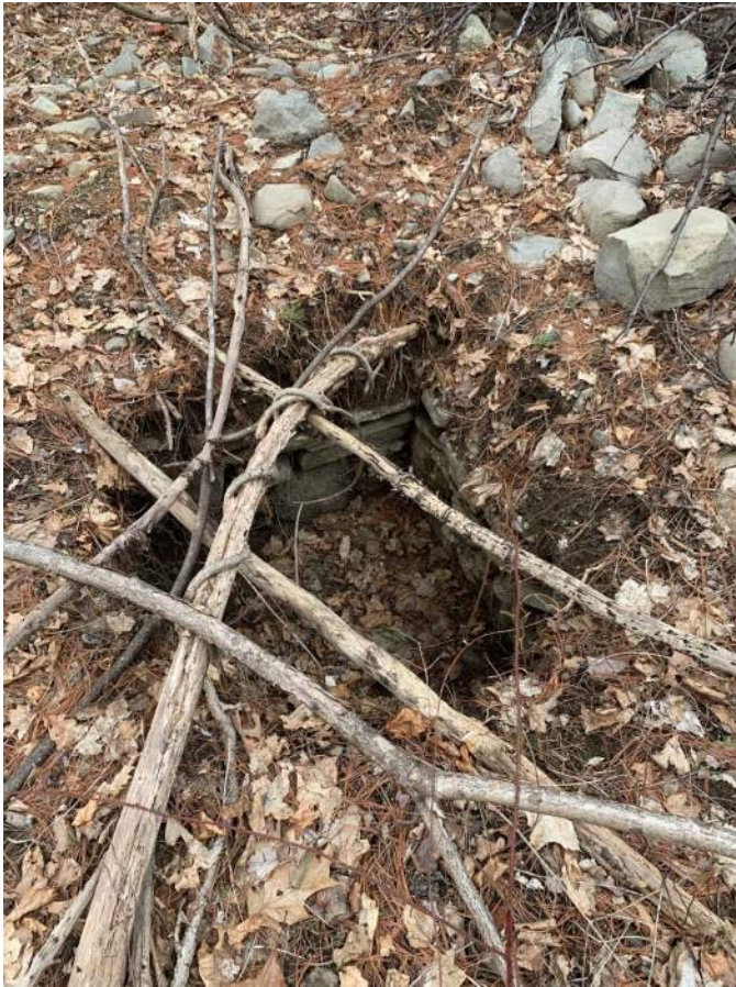
Stone lined dug well south of house
