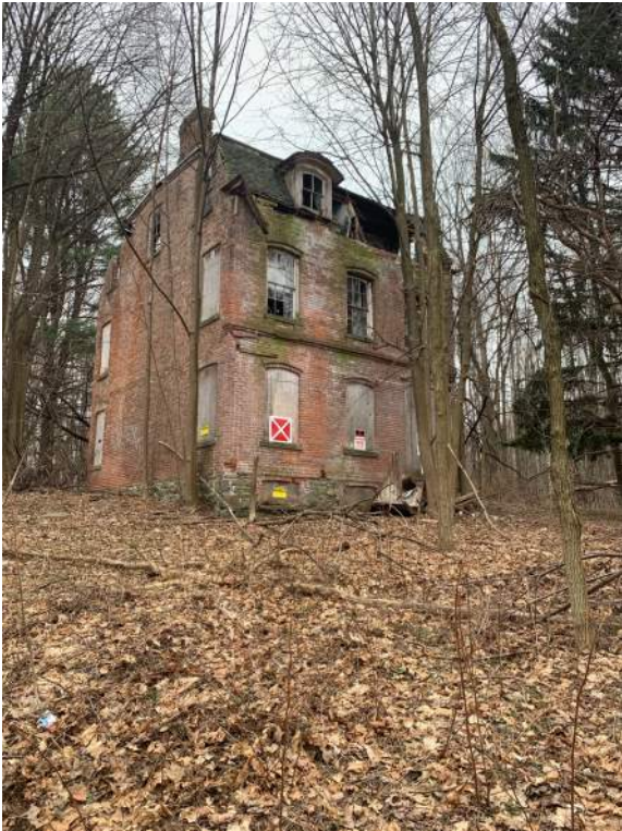
Site House North Side
